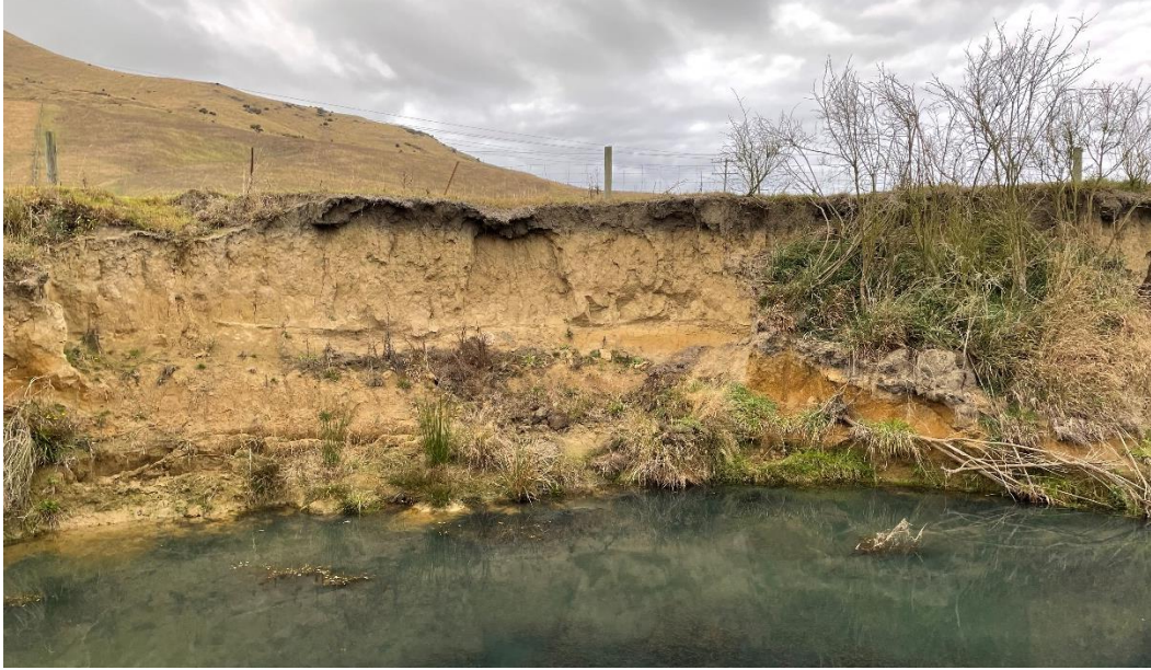
Figure 2-9: Streambank erosion in Pleasant River at FAMILTON FARM off SH1 (site Slip-Rep3), May 2022. Photo: IMG_3768.jpg, Elliot Bowie (NIWA).
