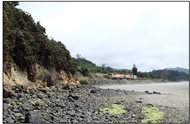
Artificial rock walls for rail infrastructure on the western margins
