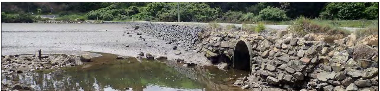
A causeway cuts across the southern end of the estuary.
