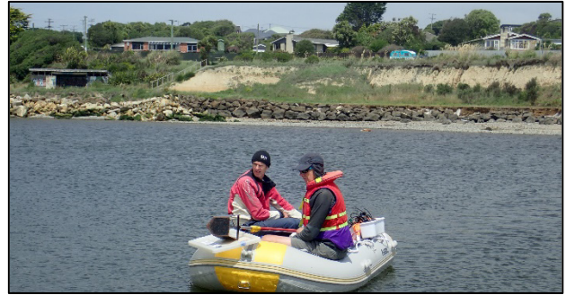
Kakanui settlement, rock wall providing erosion protection
