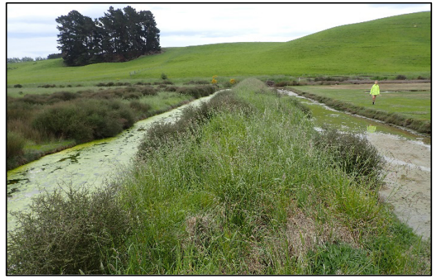
Causeway across the west arm, with water flow into the upper arm restricted by a flapgate (left farmland and right salt marsh)
