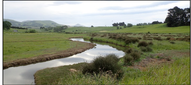
Stream input, with seawater incursion restricted by flapgates
