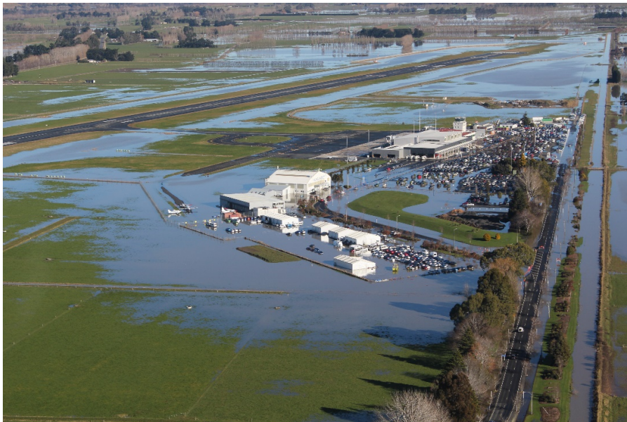
Figure 8: Dunedin Airport, flooding event 2017.
