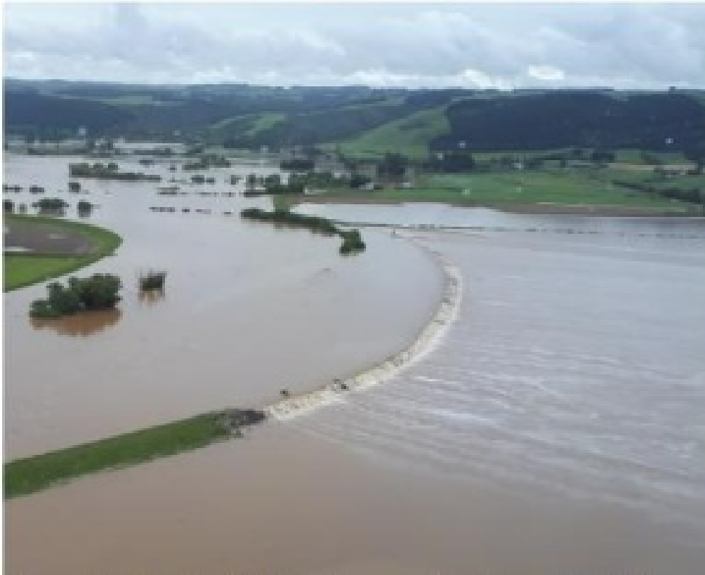
Figure 6: Riverside Spillway operating November 2018. The Taieri River is at left (looking upstream).
