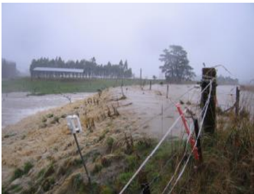
Photo 6: Image showing Contour Channel overtopping downstream of Huntly Road, April 2006.
