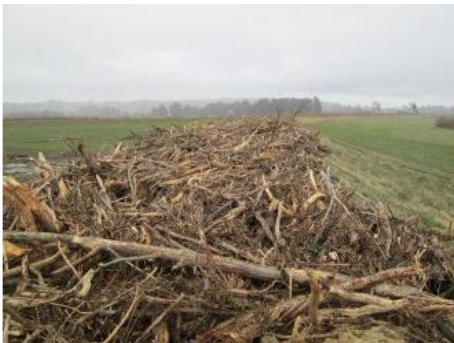
Image 10: Crest debris, Riverside Spillway, July 2017
