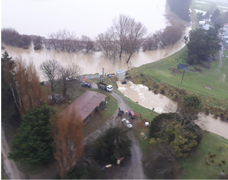
Photo 1: Image showing Mill Creek Pump Station during 2017 flood.
