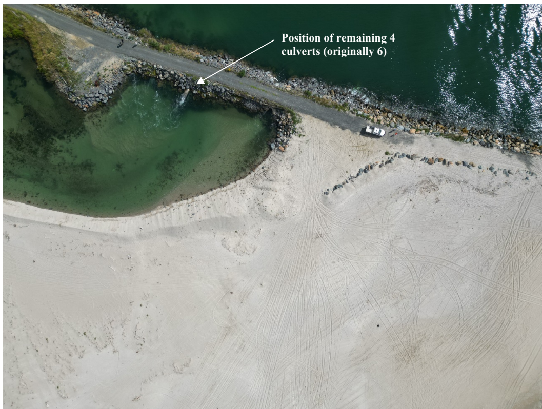
Figure 10: Section of the Training line with the remaining culverts, 19 January 2024.
