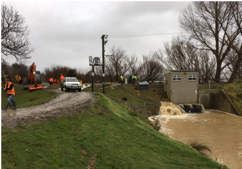
Photo 2: Image showing Mill Creek Pump Station during 2017 flood.
