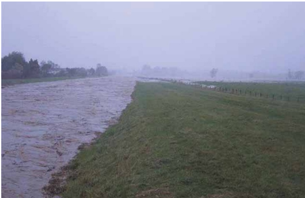
Figure 5: Gordon Road Spillway operating (April 2006).
