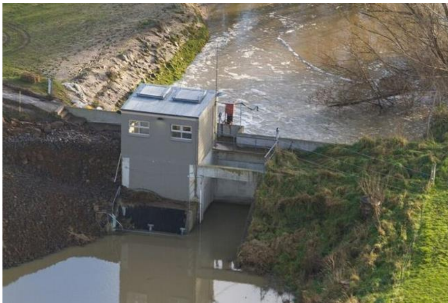
Photo 3: Image showing Mill Creek Pump Station during 2017 flood.
