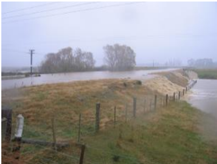
Photo 7: Image showing Contour Channel overtopping downstream of Huntly Road, April 2006.
