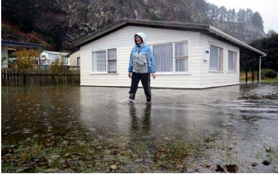
Figure 45 Water ponding on a property at Long Beach after heavy rainfall in May 2010 (source: ODT)
