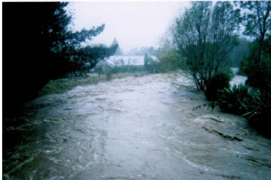
Figure 52 Waitati River close to overtopping the true left bank, downstream of the Harvey Street Bridge, April 2006
