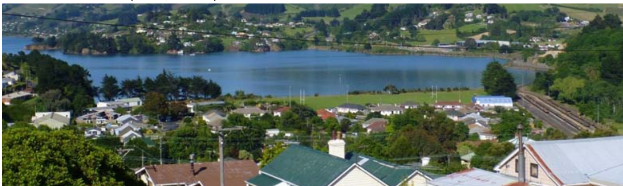
Figure 29 View to the south, showing reclaimed residential land at Port Chalmers
