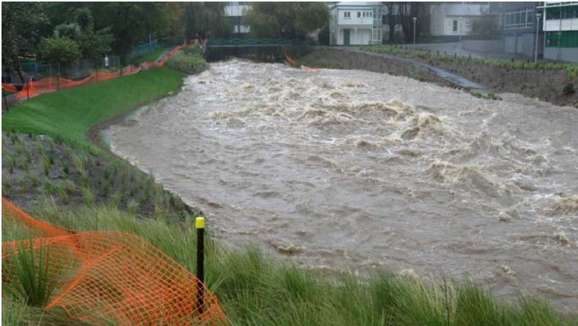
Figure 3 The Water of Leith channel, downstream of Leith Street, at approximately midday on 18 April 2014 (taken close to the peak flow on that day of 71\text{m}^3/\text{s} – see Figure 9). Works to improve the capacity of this reach commenced in 2011. Photo source: Jeff King
