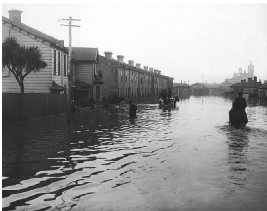
Figure 10 Floodwater from the Water of Leith ponding in Harrow Street (looking south towards the Railway Station), April 1923. The approximate location of this photo is shown in Figure 32.
