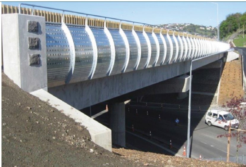
The Glen Bridge, Caversham Valley
