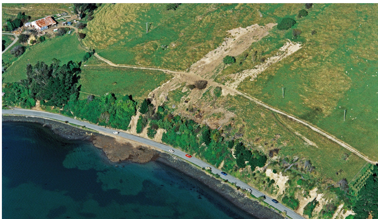
Figure 12 Surficial landslides occurred above Portobello Road, between Challis and Glenfalloch, during the March 1994 rainstorm, and generated debris flows that ran downslope, crossed the road and accumulated in Otago Harbour. The photo was taken after the debris had been cleared off the road, although the debris remains evident on the foreshore (brown) and seabed (pale). Being one of only two access roads to Otago Peninsula, this photo illustrates the potential vulnerability of this key transport route for peninsula residents. Photo: GNS Science, D.L. Homer, CN32057b, 1 May 1994.
