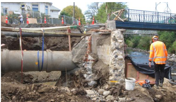
Photograph 4: Excavation at western end of St David St footbridge.
