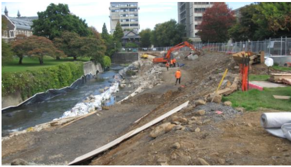
Photograph 5: Works to western side of Water of Leith.
