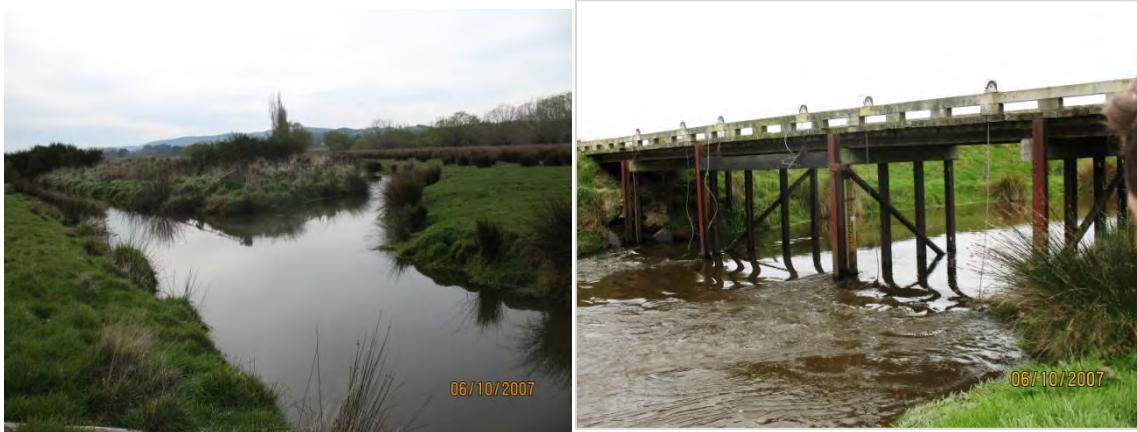
Figure 8 The left hand photo shows Stony Creek converging with the diversion channel and the right hand photo shows the Lake Tuakitoto outlet sill.
