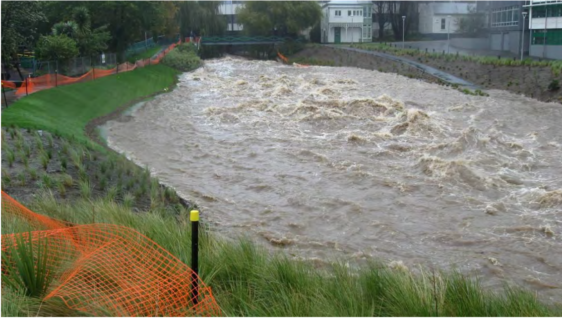
Figure 3 The Water of Leith channel, downstream of Leith Street, at approximately midday on 18 April 2014 (taken close to the peak flow on that day of 71m 3 /s – see Figure 9). Works to improve the capacity of this reach commenced in 2011. Photo source: Jeff King.
