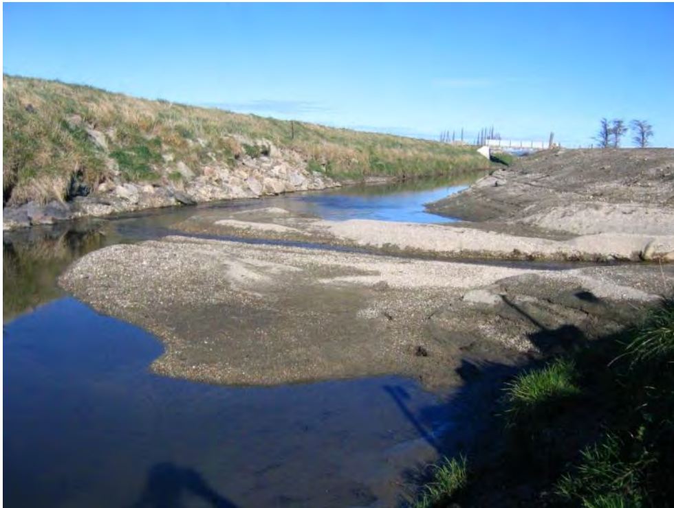
Figure 9 Deposition of gravel in the Contour Channel from a tributary hill stream
