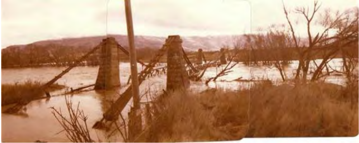
Figure 42 Taieri River at Sutton Bridge, during the June 1980 flood
