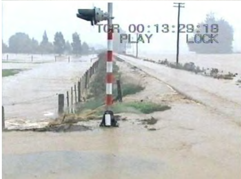
Figure 22 Water ponding behind the Taieri Gorge Railway, 26 April 2006
