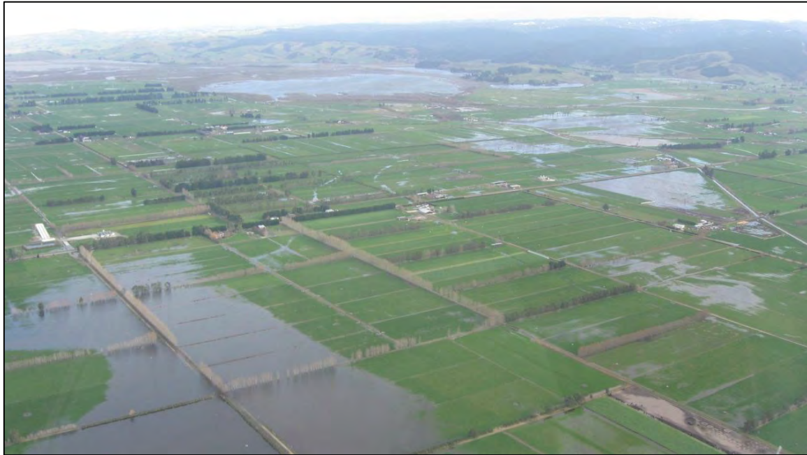
Figure 4 Aerial view of ponding on the West Taieri Plain, resulting from internal runoff from Area 1A and 1B during heavy rainfall in June 2013 (195mm over 8 days at the Riccarton Road rain gauge). Lakes Waipori and Waihola can be seen in the distance.
