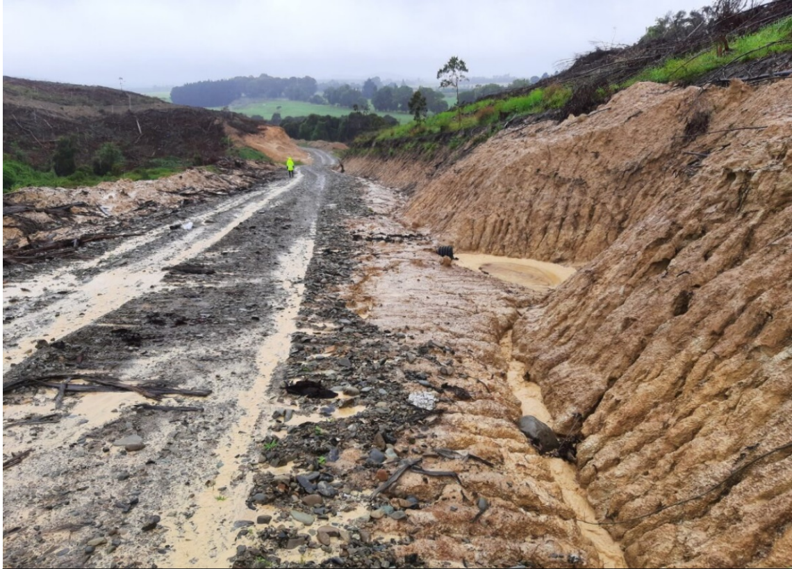
Image 2: Downhill of haul road: (Right side) Water table with stormwater containing substantial amounts of sediment within it. A sediment trap is located before a culvert pipe before discharging to the receiving environment – sediment exposed above the waterline would suggest this trap required maintenance
