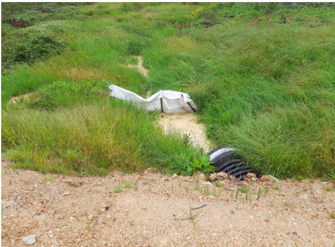
Image 3: Discharge point from culvert: Silt fence is placed at the outlet as further stormwater control – clarity of water is still poor beyond the silt fence.
