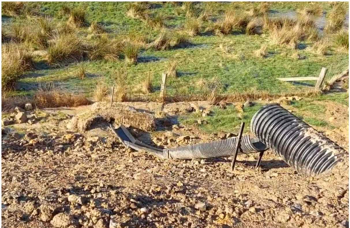
Image 8: Stormwater flume discharging to a sediment trap with hay bales – sediment controls have been inundated with sediment and is overflowing.
