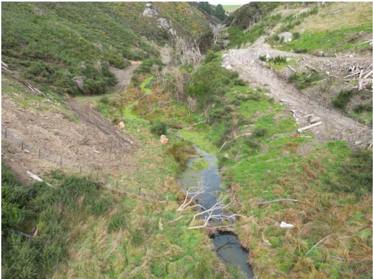
Image 13: Watercourse between cable hauling points - Tracking from activities has not been stabilised or controls put in place
