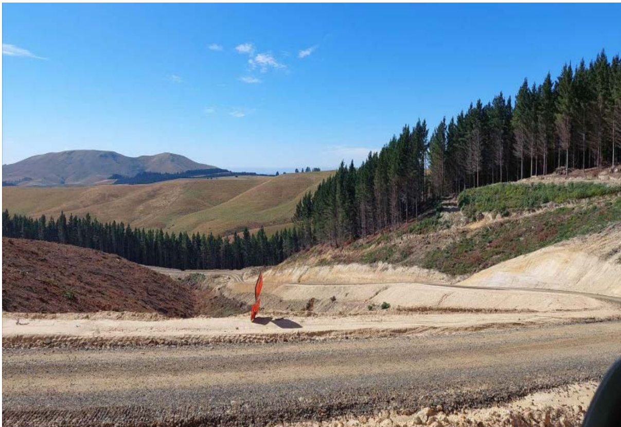
Image 6: Haul road up-hill from sediment discharge: Cut faces from road construction are battered and compacted, side-cast/fill material has been compacted and appears to be placed on
