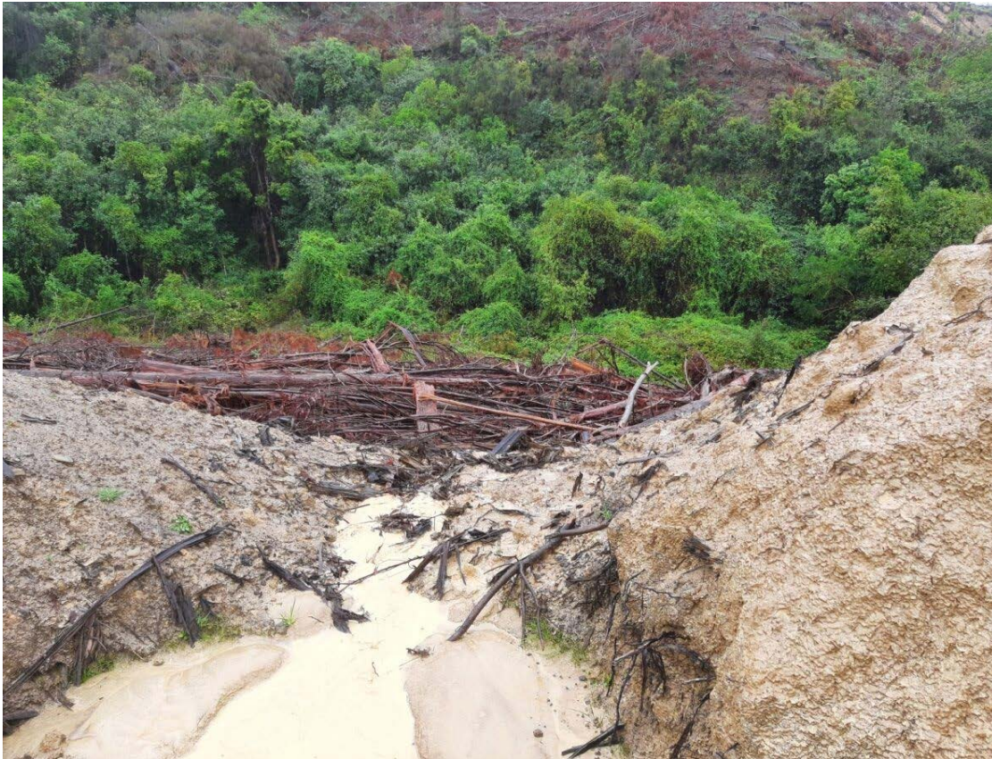
Image 4: Discharge point from Haul road's water table: Flow is being dispersed into slash as a filtration method and into native forest
