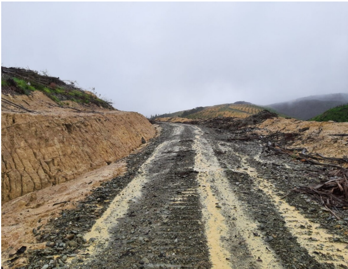
Image 1: Haul road within the forestry block: (Left side) material from road construction has been compacted but has not achieved adequate stability due to erosion. (Right side) Spoil material is sitting on side of road un-stabilised; slash appears to have been used as mulch in some areas but ineffective.
