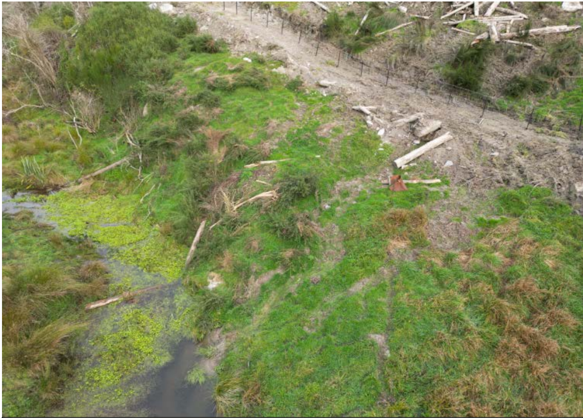
Image 14: Sediment running into river due to no stabilisation and controls
