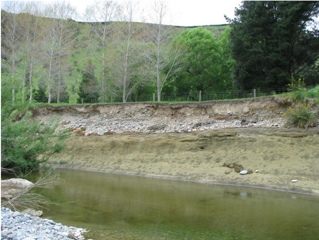
Figure 8-Area of active bank erosion on the North Branch of the Waianakarua River (upstream of SH1), photo taken looking upstream, October 2013
