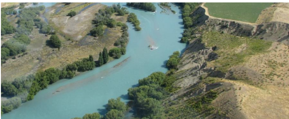
Figure 22. View of the Clutha River/Mata-Au, looking downstream and showing erosion of the true right bank (point 4 on Figure 15). Photo taken 15 January 2013.
