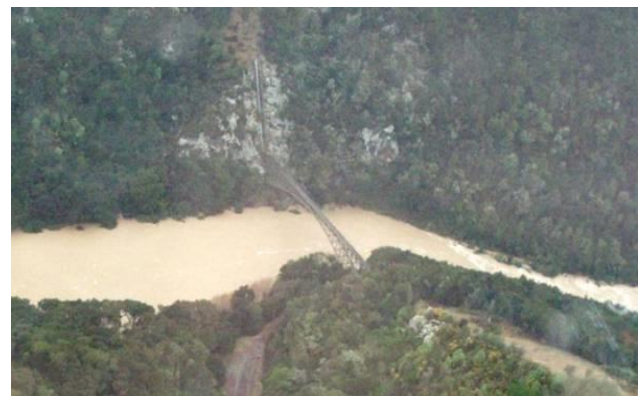
Taieri Bridge carries critical water pipes for Dunedin
