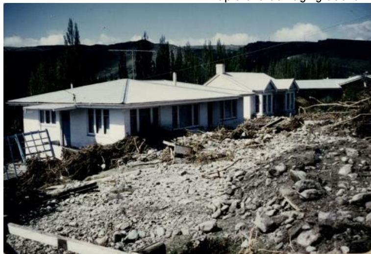
Sediment and debris cover the lower portion of the Reservoir Creek alluvial fan, Roxburgh, following heavy rain on 16 October 1978
