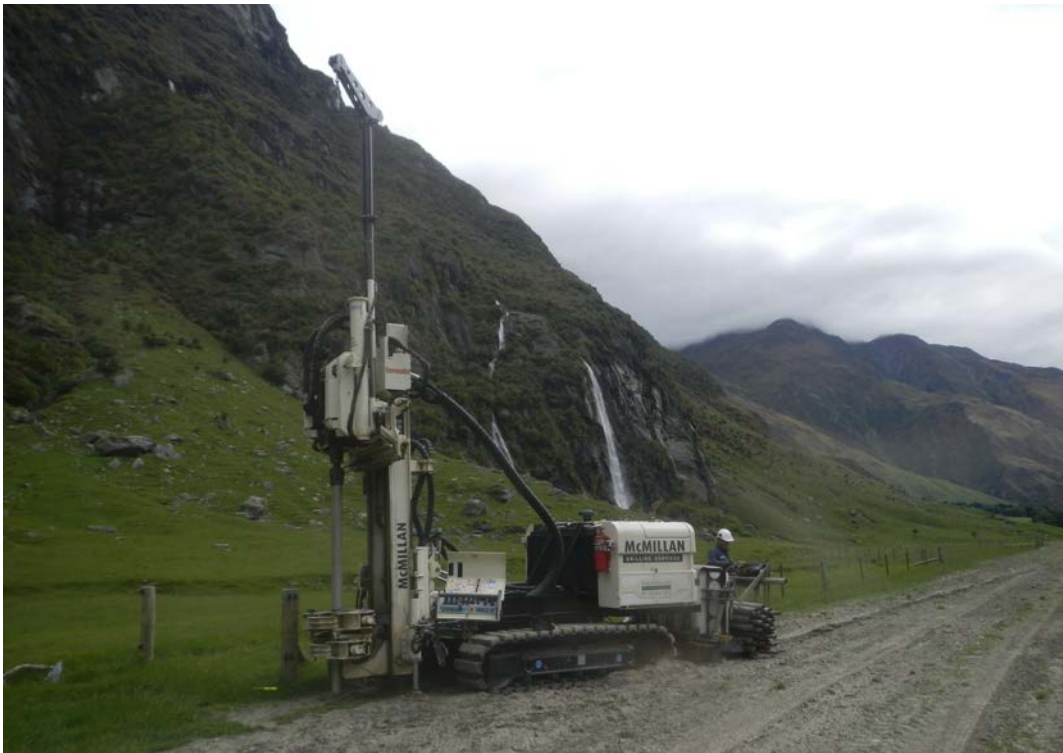
Figure 4. Drilling rig installing groundwater monitoring bores.
