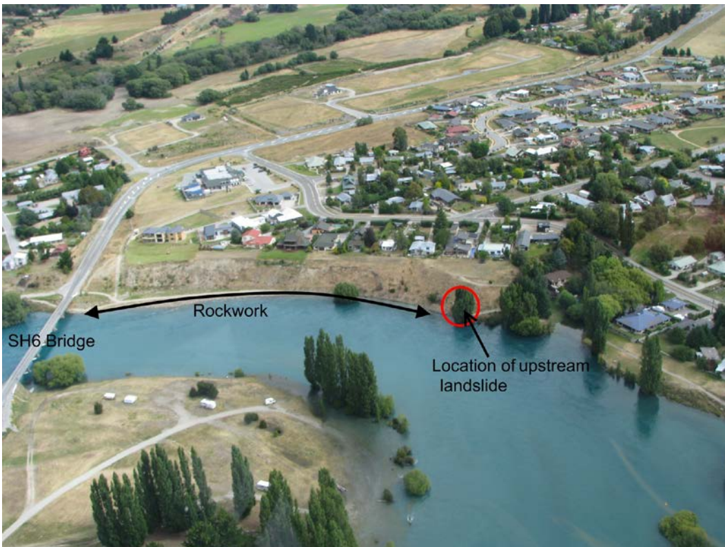
Figure 7. Aerial view showing extent of the ORC's rockwork, and the location of the upstream landslide (taken during a period of high flows in the Clutha River, January 2013).
