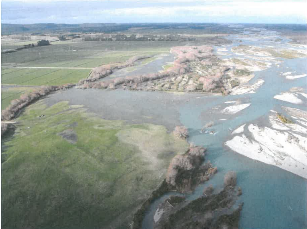
Photo 1-3: Farm encroachment onto berm lands
