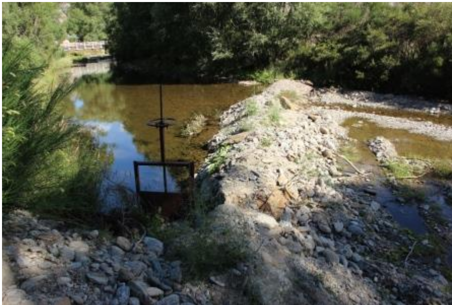
Figure 42 Gravel bund downstream of Styx-Patearoa Rd - 16 th January
