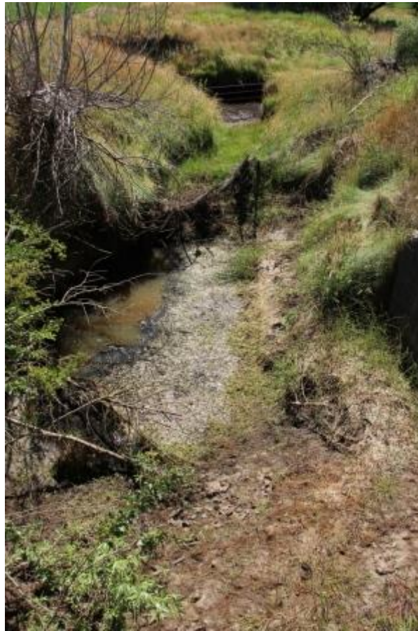
Figure 31 Isolated pools upstream of the Puketoi-Highfield Rd bridge - 16 th January
