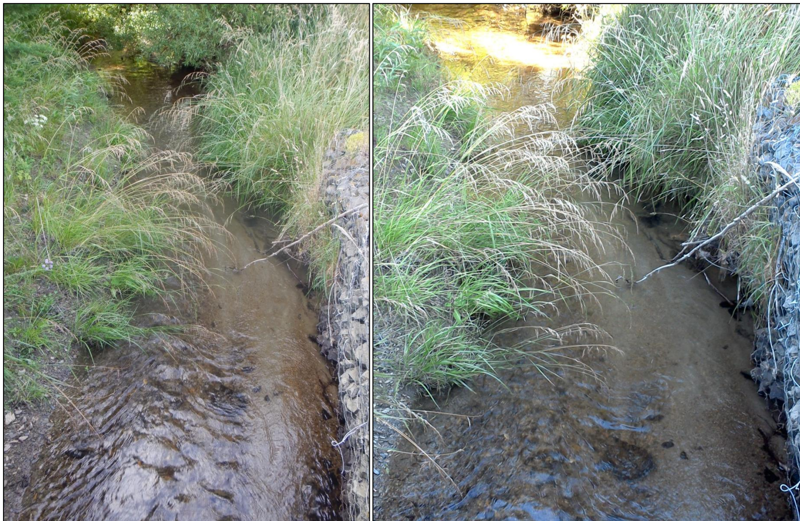
Figure 10 Rock Creek SH87 on January 14 th (left) and 16 th January (right)
