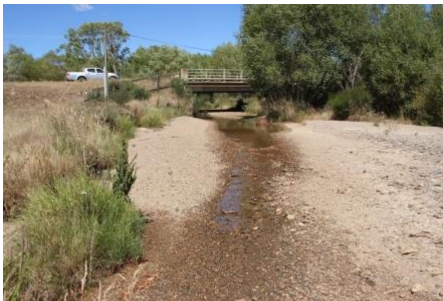
Figure 24 Beginning of dewatered reach in the Pig Burn 40 m downstream of the Patearoa-Waipiatā Rd Bridge - 16 th January
