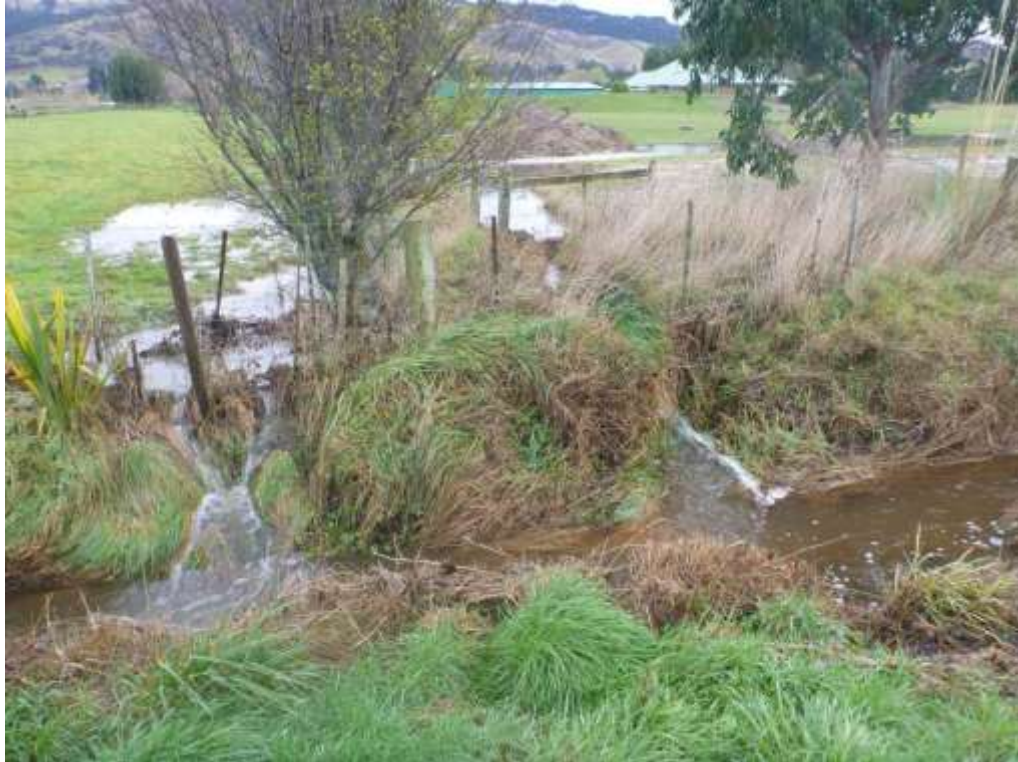
Figure 42. Example of overland flow path conveying runoff from the hill catchments to an ORC drain between Riccarton Road and Gordon Road – 4 June 2015
