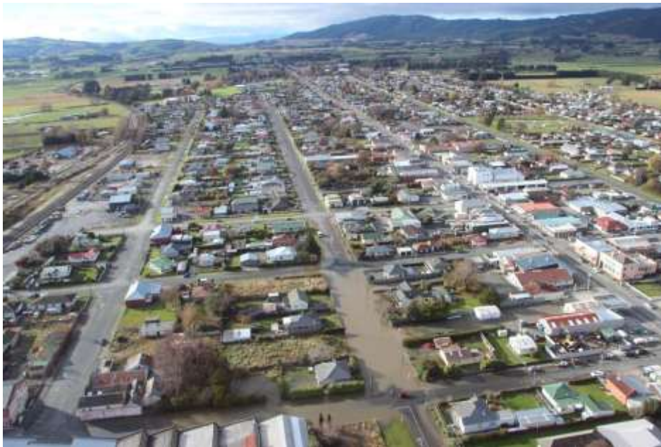
Figure 49. Aerial view of floodwater on Ajax Street (centre) Milton, with Union Street (SH1) to the right, 4 June 2015
