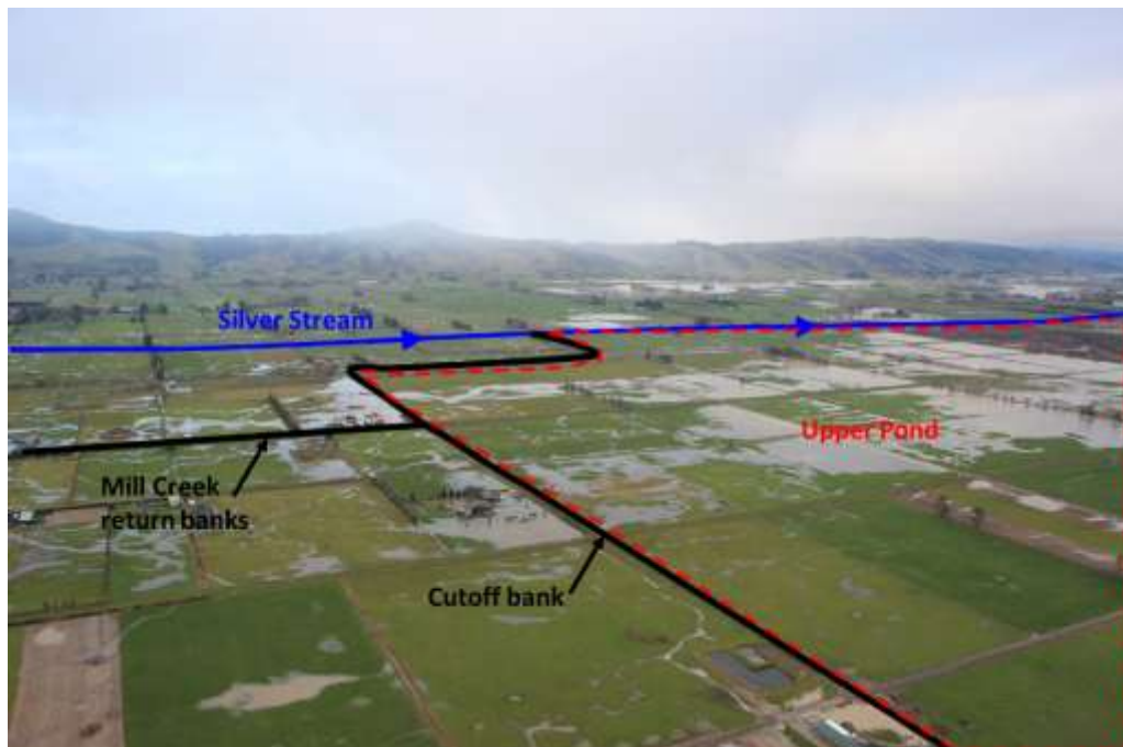
Figure 40. Ponding behind the Cutoff Bank, view is towards the south – 4 June 2015
