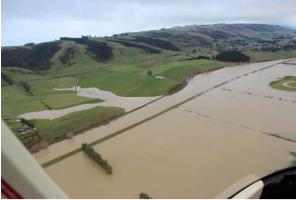
Figure 44. Ponding in the Lower Pond (note the overtopping of the Owhiro Stream true right bank) and at the flanks of the coastal hills – 4 June 2015
