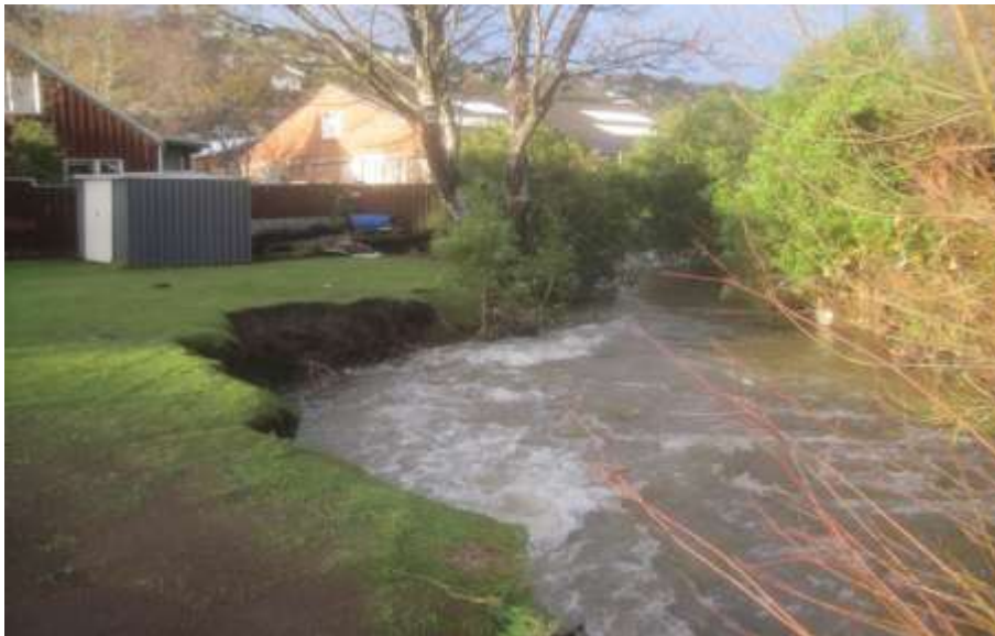
Figure 29. Bank erosion alongside Lindsay Creek at Kelvin Road, 4 June 2015
