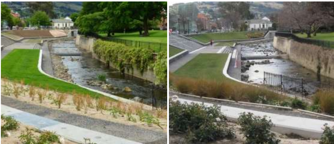
Figure 25. Water of Leith before and after – looking upstream from near the Staff Club. Note the loss of some riprap on the true right bank.
