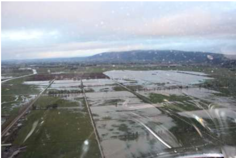
Figure 38. Ponding in the Upper Pond, view is towards the southwest – 4 June 2015
