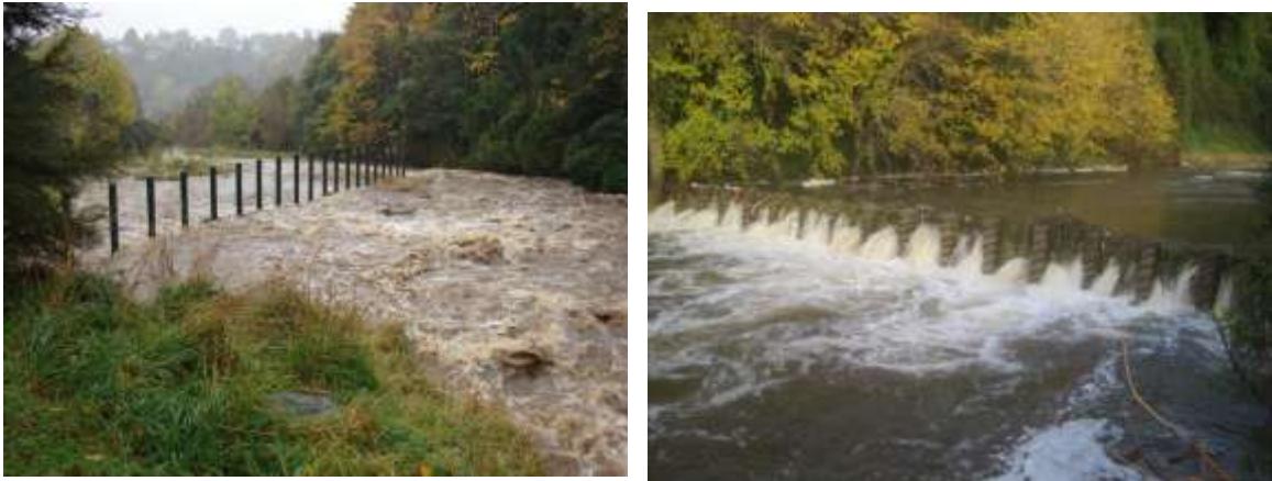
Figure 26. Water of Leith debris trap at Malvern Street (left) and Woodhaugh Street boulder trap (right) during the event, 3 June 2015
