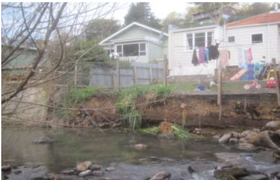
Figure 30. Bank erosion alongside Lindsay Creek at Norwood Street, 4 June 2015
