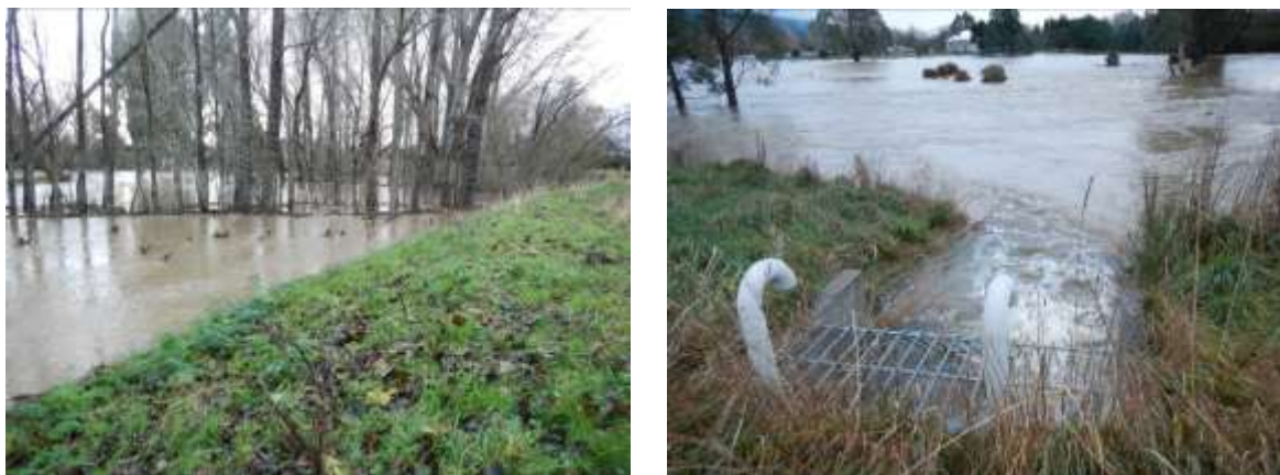
Figure 47. The floodbank (left) and pump station outlet (right) at Milton, downstream of SH1, 3 June 2015
