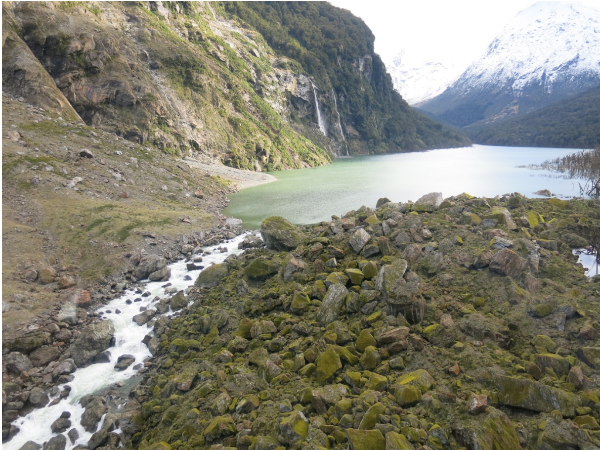
Figure 31. View of the Young River Landslide Dam. A landslide in August 2007 dammed the Young River to a height of 70m, and formed a ~1.5 km long lake. (May 2015)
