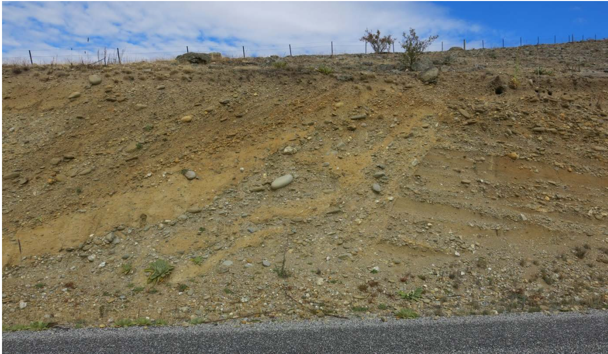
Figure 23. Road cut along Mt Pisa Road showing faulted alluvium and glacial till units along the Pisa Fault Zone. The gravels, assessed as outwash deposits, are associated with the Lindis glacial advance (~430,000 years old).
