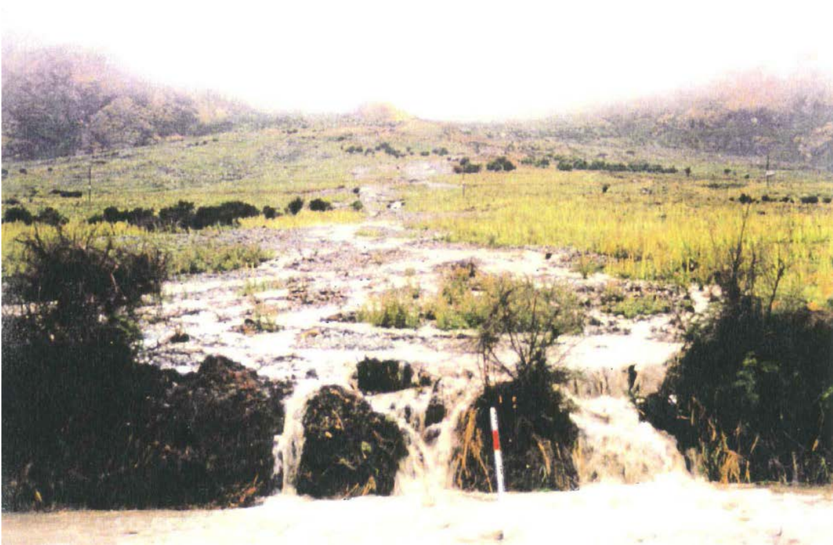
Figure 44. Active alluvial fan and debris deposition in February 1994 as seen from SH6 looking towards the Remarkables. Gravel was deposited across SH6. These fans have potential to become more active if the headwaters are inundated with sediment following an earthquake. Photo from Cunningham (1994).
