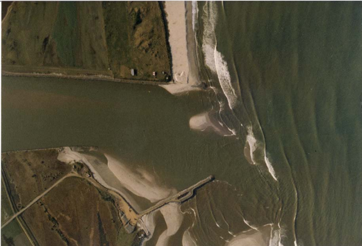
Figure 4.4 Koau Mouth works- June 1983 (during construction).
