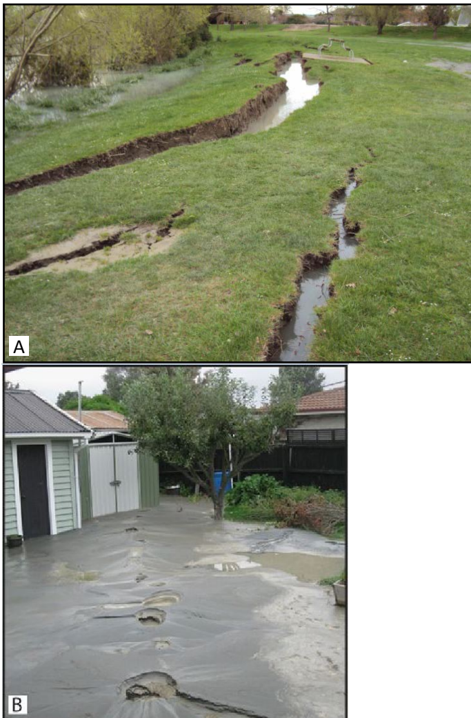
Figure 5.3 a) Lateral spreading on the true-left bank of the Kaiapoi River, after the Christchurch magnitude 6.3 earthquake. b) Sand boils in Avonside after the Christchurch earthquake in February 2011 (after Quigley et al. , 2013).
