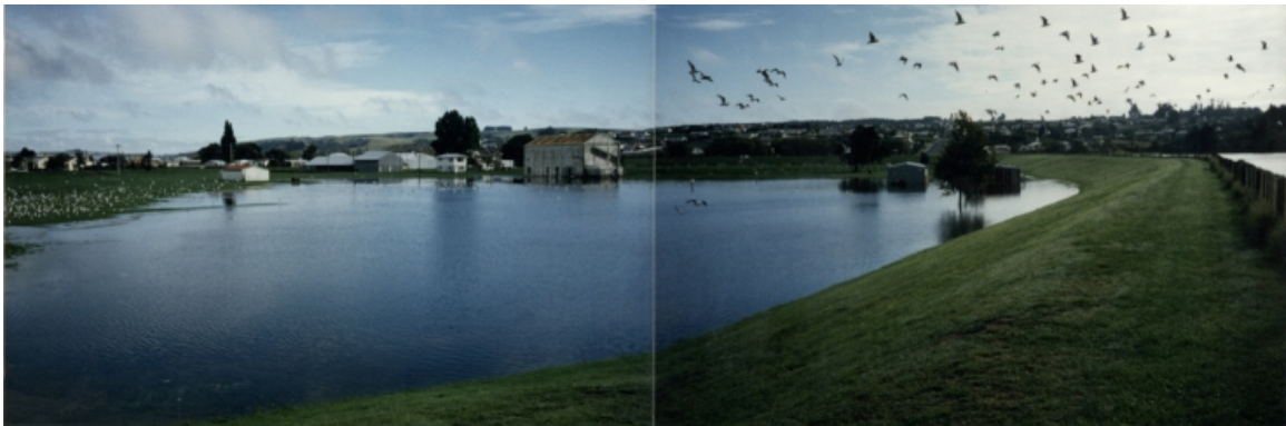
Figure 4.18 Localised ponding due to seepage coming from the relief wells on the landward side of the floodbank at the Balclutha Showgrounds during the March 1987 flood event ( 2300 \text{ m}^3/\text{s} at Balclutha).
