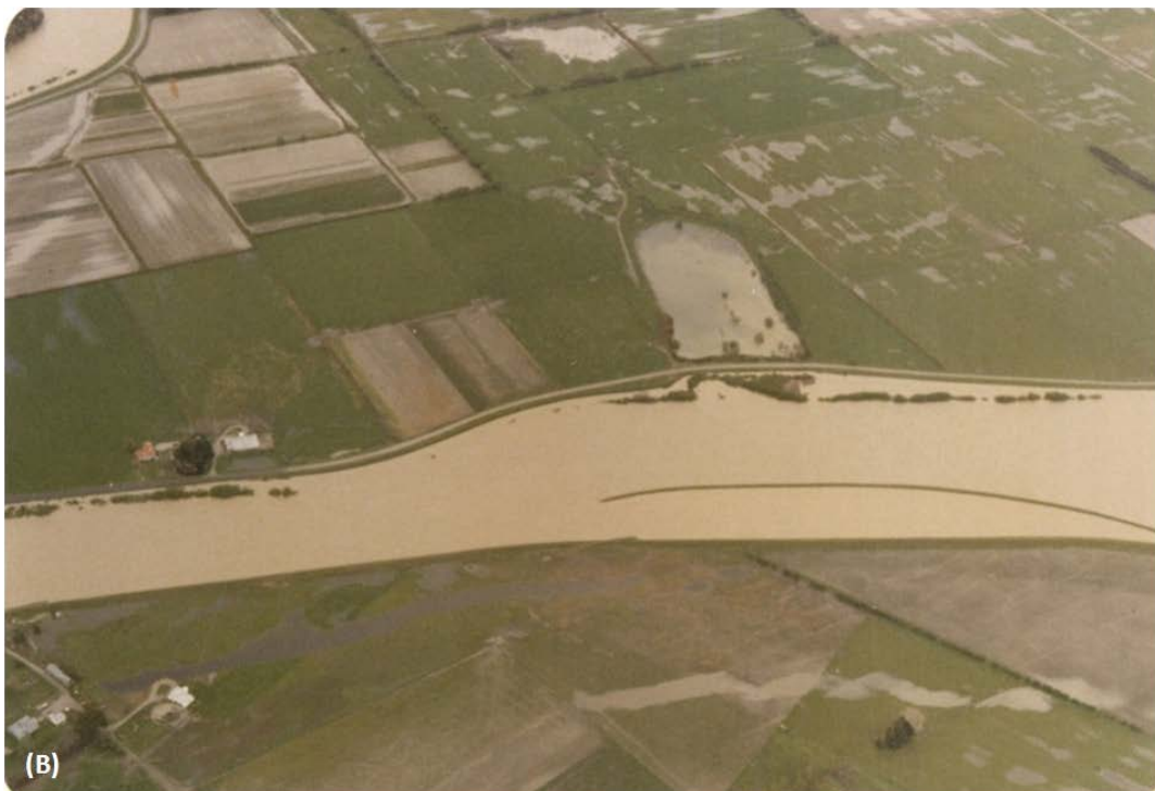
Figure 4.25 Location of Weirs Gap (A) and Weirs Gap during the October 1978 flood event (B). Note the water from seepage under the floodbank ponding on the landward side of the floodbank in the balancing pond.
