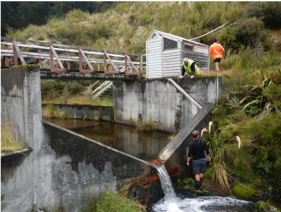
Figure 2. Picture showing v-notch flow recording weir and site shed. Continuous turbidity monitoring sensors and automatic water samplers are located directly upstream of the concrete infrastructure to the left of the picture.
