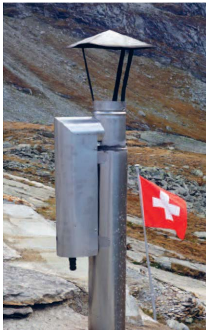
Figure 2. An Oeko Tube installed on a chimney uses the principles of electro-static precipitation to “filter” particulates out of the airstream before they are released into the atmosphere.
