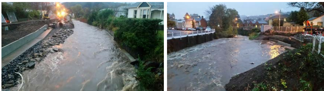
Figure 1: Dundas Street to St David Street Reach of the Water of Leith during the rain event on 23 May 2016. Photos are taken at 8.15am approximately 8 minutes after the flow peaked.
