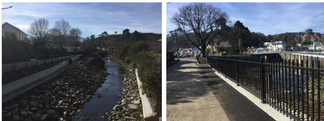
Figure 1: Dundas Street to St David Street Reach of the Water of Leith, St David Street pathway (left) and looking towards Dundas Street (right), on 19 August 2016.
