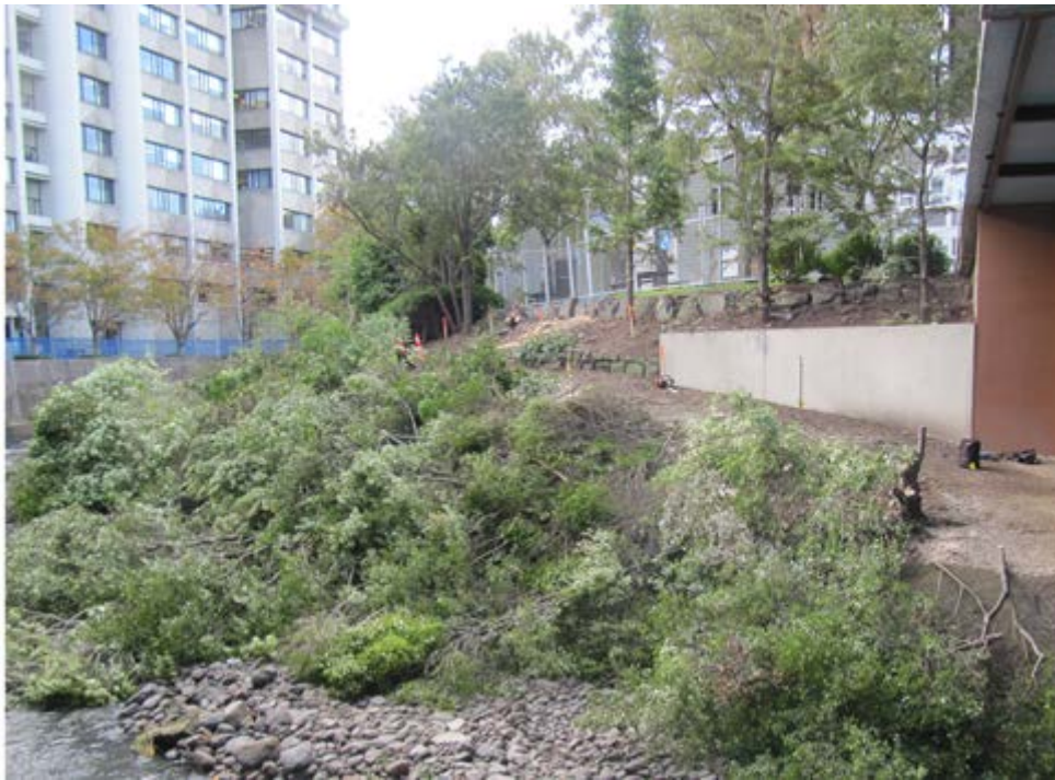
Figure 2: Left bank vegetation clearance in Memorial Garden on 19 April 2017. Selected trees are being retained and incorporated into the scheme works as requested by the University of Otago
