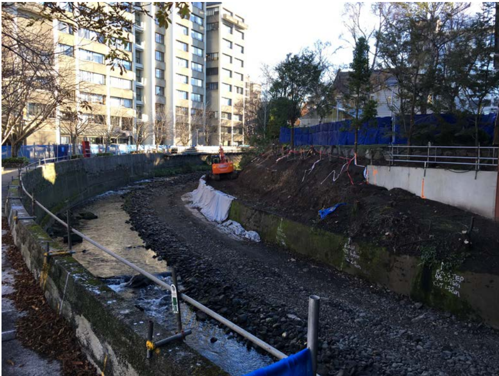
Figure 1 Water of Leith left bank excavation immediately upstream of ITS building.
