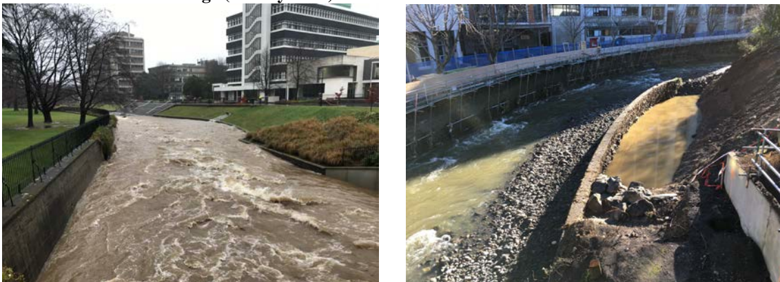
Figure 4: Leith Flood Protection Scheme following the flood event on 21 – 22 July 2017.
