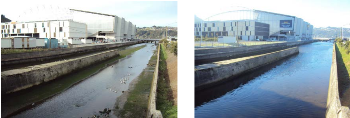
Figure 2: Water of Leith at low tide, before (left) and after (right) the construction of weirs downstream of ANZAC Street in 2011.
