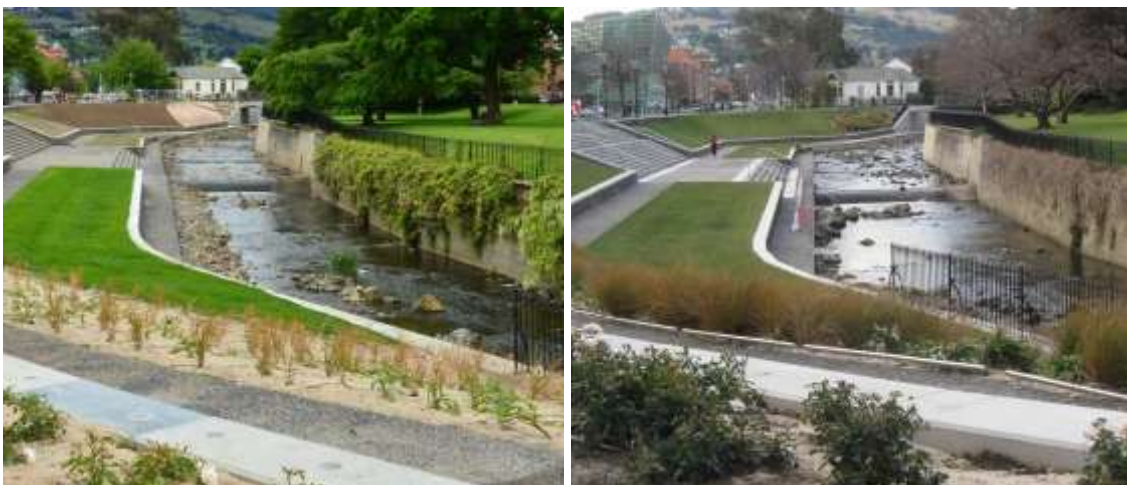
Figure 27. Water of Leith before and after: Looking upstream from the University of Otago Staff Club. Note the loss of some riprap on the true-right bank.
