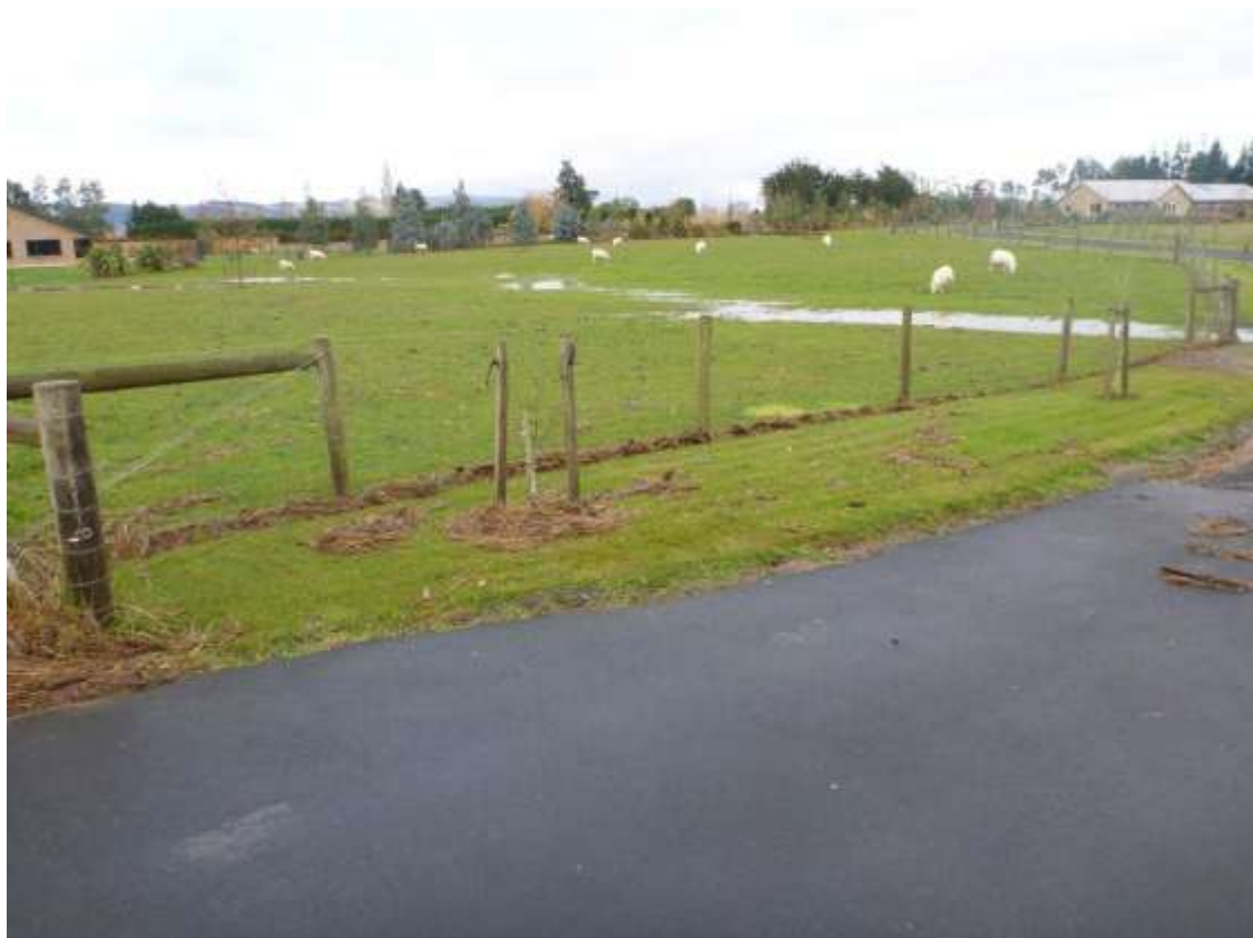
Figure 43. Debris marks indicative of overland flow and ponding in the vicinity of Wyllies Crossing – 4 June 2015
