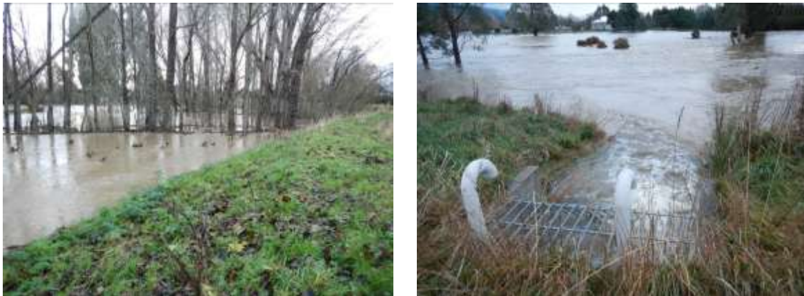
Figure 49. The floodbank (left) and pump station outlet (right) at Milton, downstream of SH1, 3 June 2015
