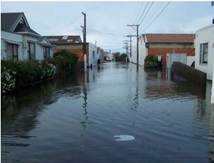
Figure 14. Ponding of surface water on Bradshaw Street, South Dunedin, 4 June 2015
