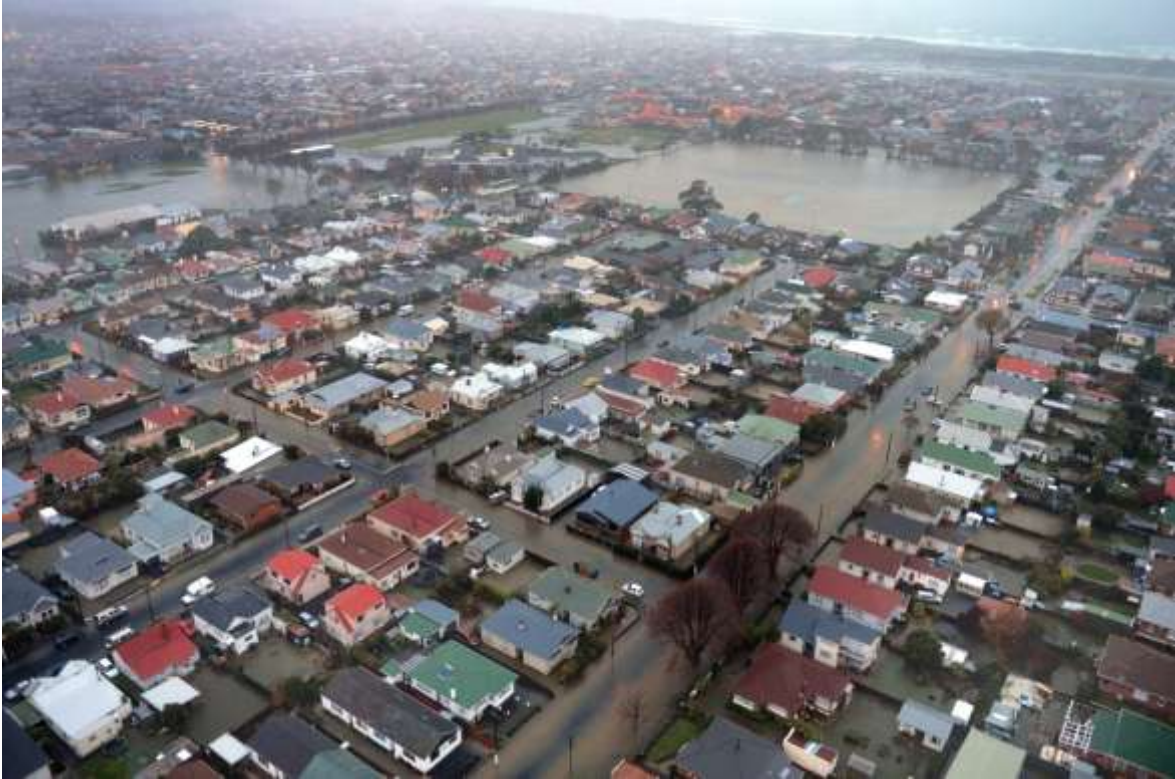
Figure 10. View of the South Dunedin area, looking southeast from near Forbury Corner, towards Tonga Park and St Kilda. Photo taken late afternoon on 3 June 2015 (courtesy Otago Daily Times).
