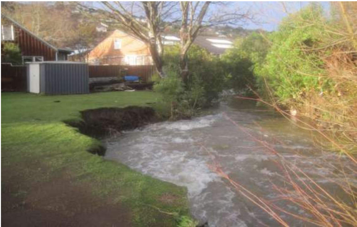
Figure 31. Bank erosion alongside Lindsay Creek at Kelvin Road, 4 June 2015
