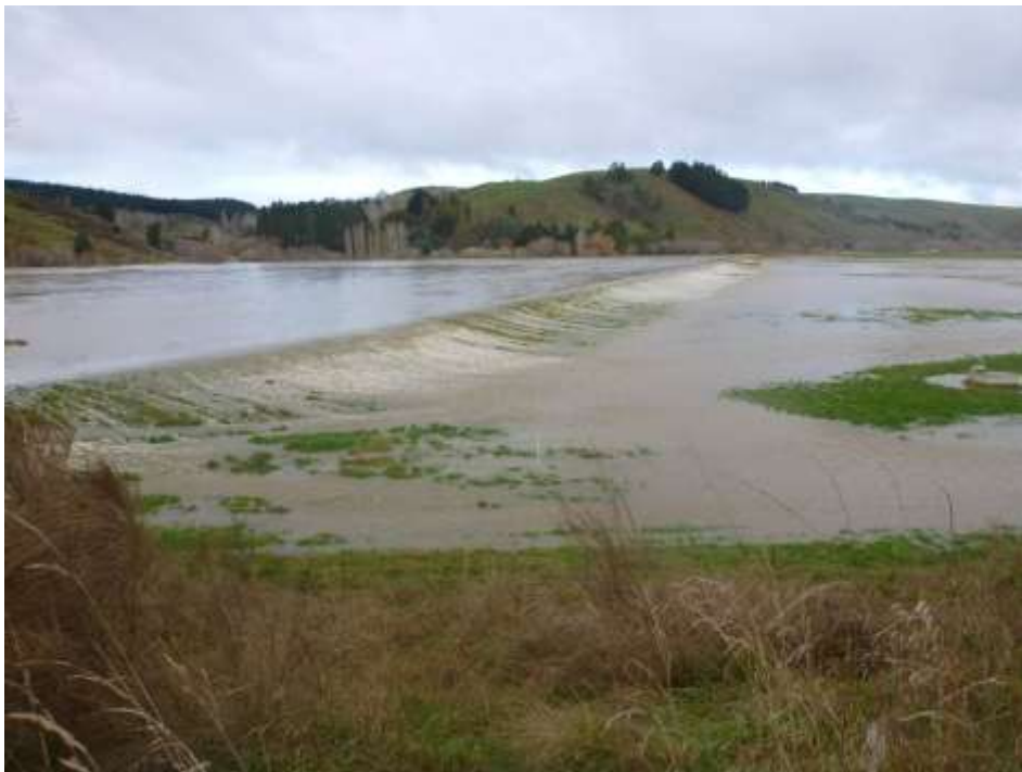
Figure 38. Henley spillway (downstream of Otokia) operating – 4 June 2015 11.45am
