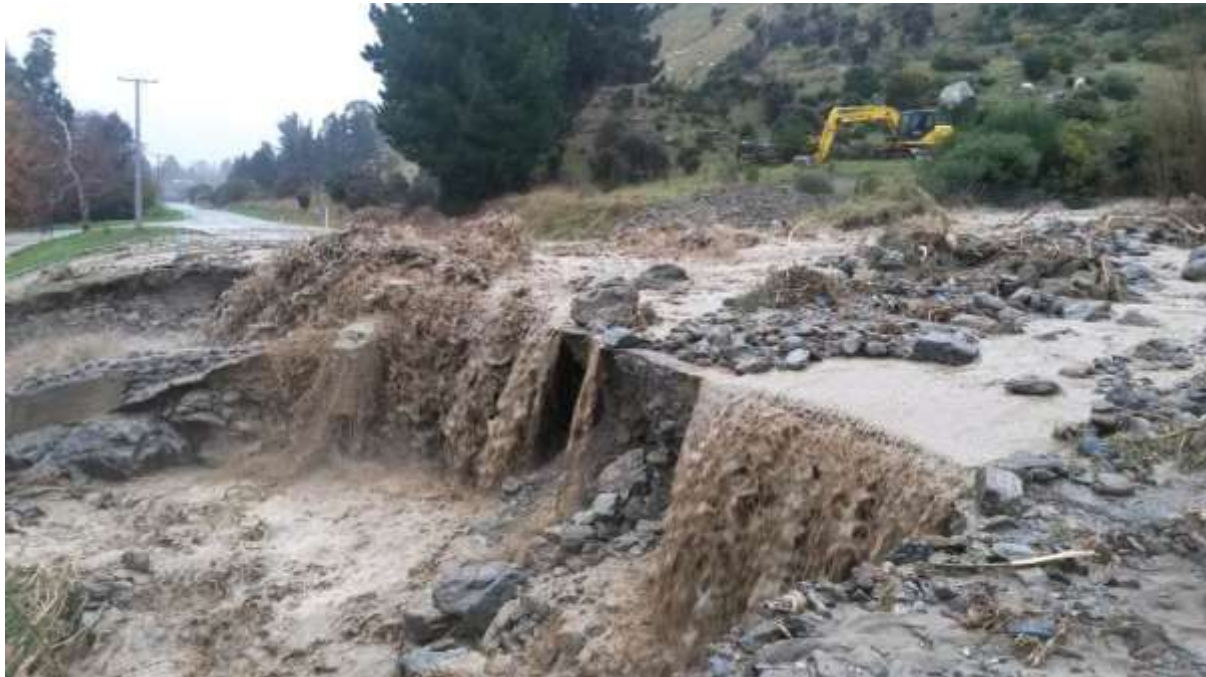
Figure 53. Flooding at Black Jacks Creek at SH8, 3 June 2015
