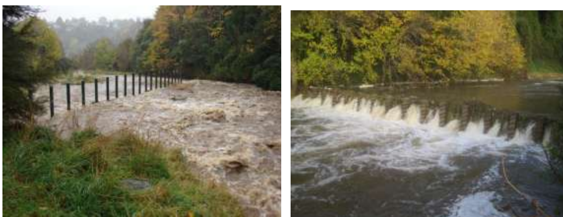
Figure 28. Water of Leith debris trap at Malvern Street (left) and Woodhaugh Street boulder trap (right) during the event, 3 June 2015
