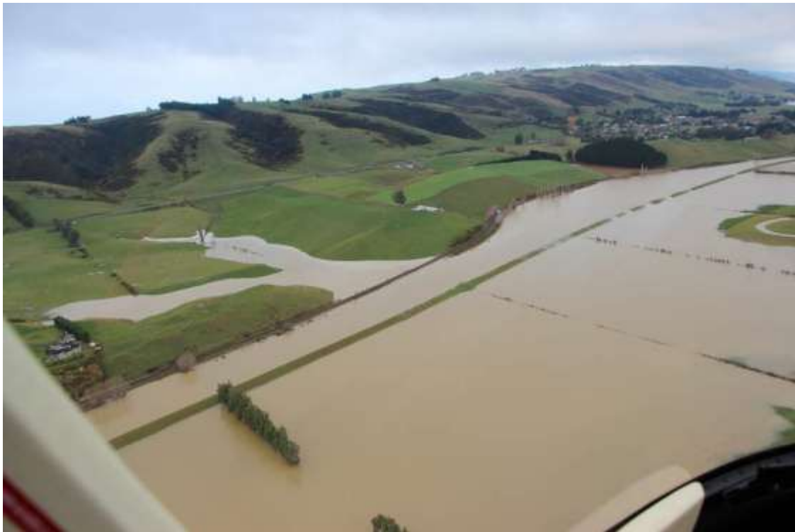
Figure 46. Ponding in the Lower Pond (note the overtopping of the Owhiro Stream true- right bank) and at the flanks of the coastal hills – 4 June 2015
