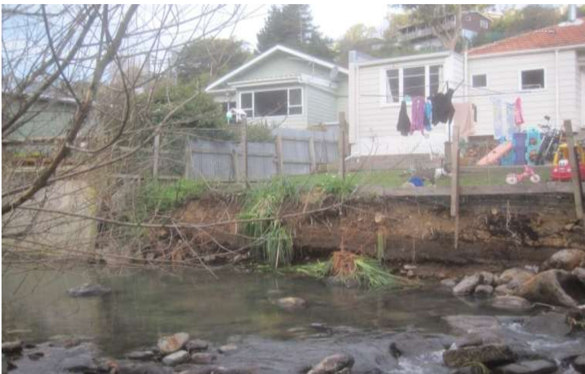
Figure 32. Bank erosion alongside Lindsay Creek at Norwood Street, 4 June 2015
