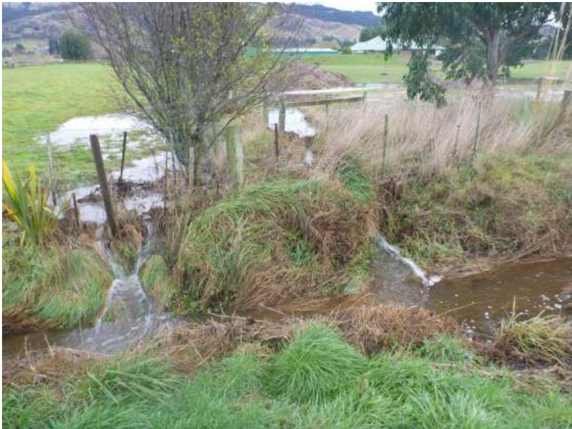
Figure 44. Example of overland-flow path conveying runoff from the hill catchments to an ORC drain between Riccarton Road and Gordon Road – 4 June 2015
