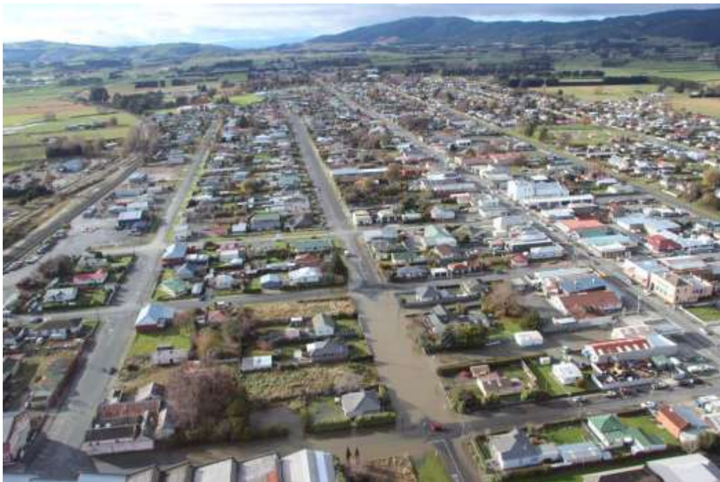
Figure 51. Aerial view of floodwater on Ajax Street (centre) Milton, with Union Street (SH1) to the right, 4 June 2015
