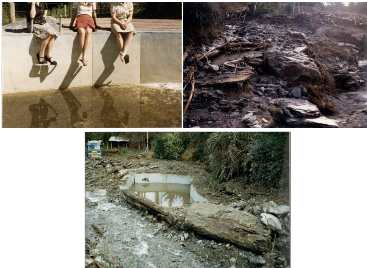
Figure 10.8 Photographs of a swimming pool on the Brewery Creek alluvial fan. Top left: Pool before May 1986, showing depth with respect to figures. Top Right: Pool filled with debris, following the storm event of May 1986. Bottom: Excavated pool after the May 1986 flood event; Brewery Creek flows to the immediate left of the pool.
