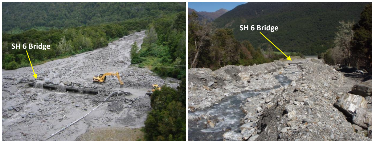
Figure 1.2 Pipson Creek in March 2004 (left), looking upstream, and November 2008 (right), looking downstream. In the left image, the creek has aggraded, so that the channels are migrating laterally outside of the channels low-flow banks; the hydrographic apex is located upstream and out of sight. In the right image, excavation and channel contouring has confined the channel to a single-thread channel, far beyond the state highway; the hydrographic apex is located near the confluence with Makarora River in this image.
