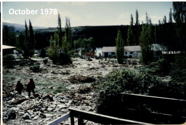
Figure 12.7 Top: Reservoir Creek at SH 8 after the October 1978 storm event, compared to March 2011. Large volumes of debris blocked the state highway in 1978 and impacted residential property. Bottom: Reservoir Creek, looking upstream (left) and downstream (right) of SH 8 in October 1978. Large volumes of debris are evident in both images.
