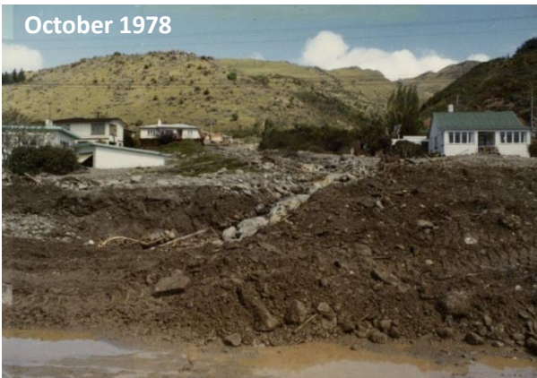
Figure 12.7 Top: Reservoir Creek at SH 8 after the October 1978 storm event, compared to March 2011. Large volumes of debris blocked the state highway in 1978 and impacted residential property. Bottom: Reservoir Creek, looking upstream (left) and downstream (right) of SH 8 in October 1978. Large volumes of debris are evident in both images.
