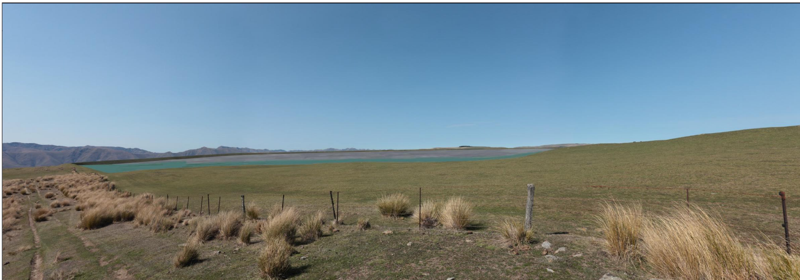
Photopoint 03a - Back Road Track (Showing tailings dam at 90% complete) - After (Textured)
