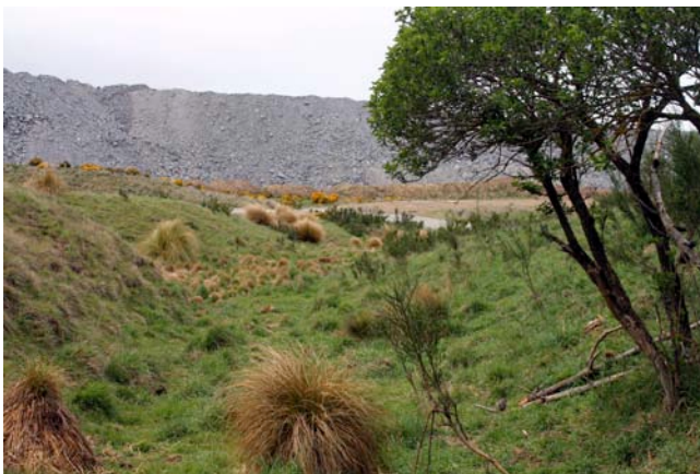
Figure 4 Looking downstream in Waikouaiti River North Branch tributary 1 to the face of Frasers East Waste Rock Stack, with dry channel at base of gully.
