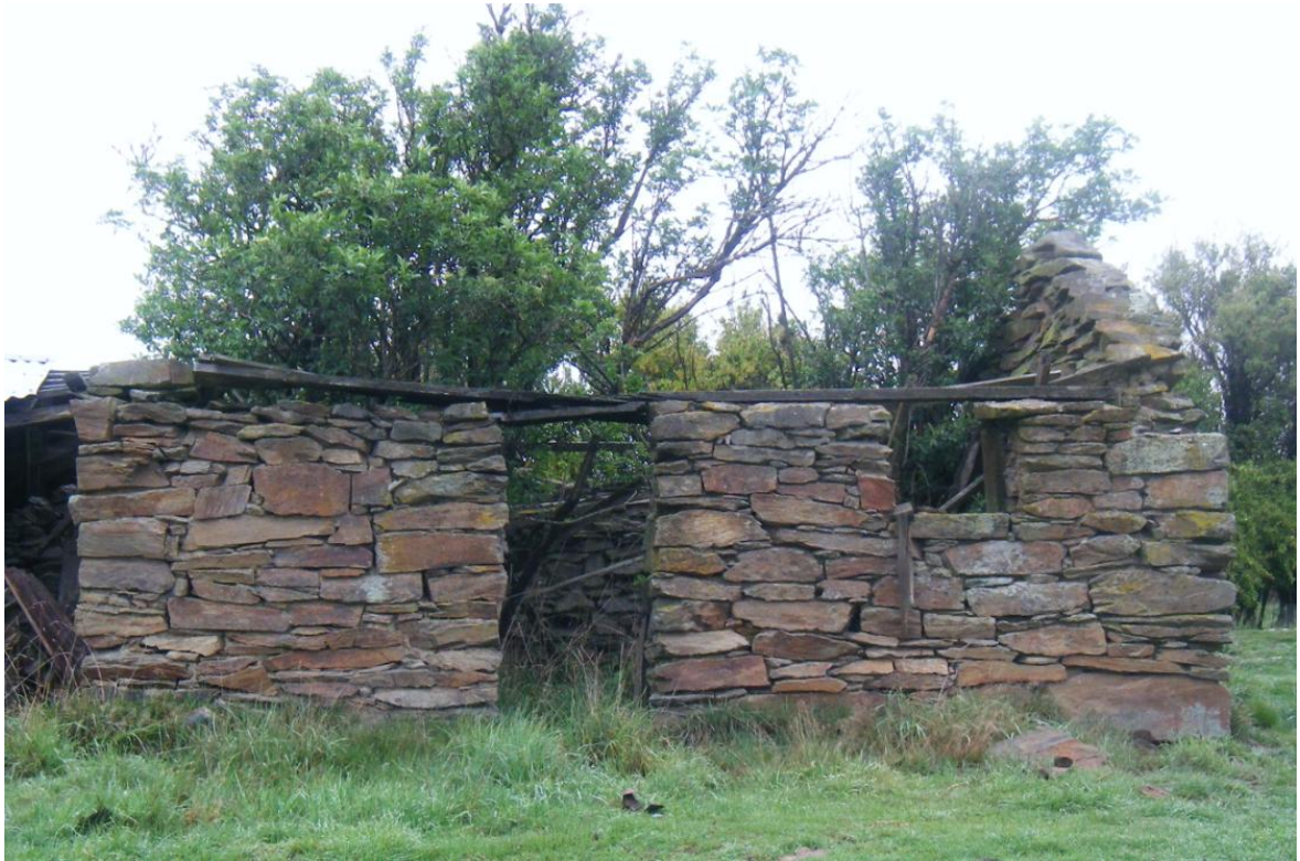
Figure Twenty Four View of front (north) face of cottage – reported to have been built in the late 1870s
