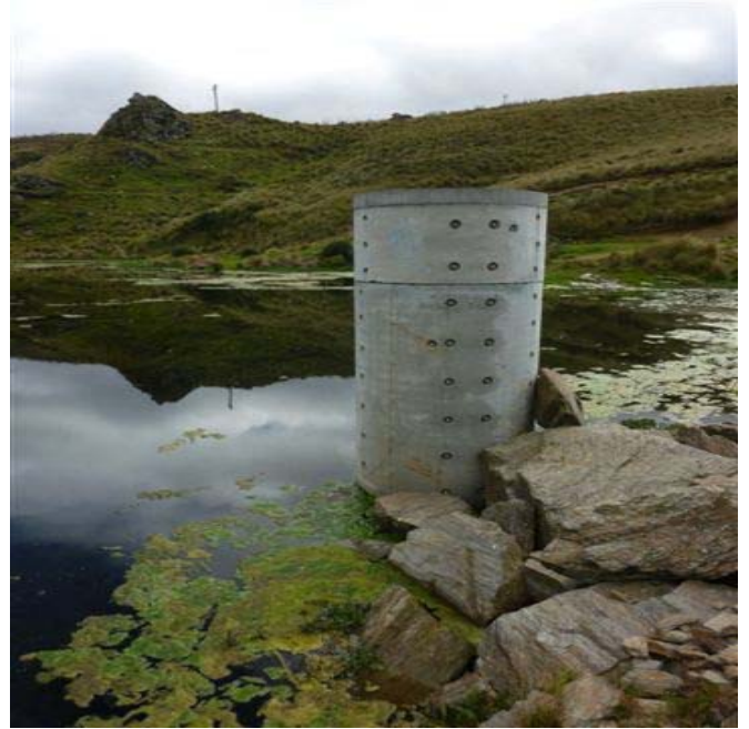
Plate 6. Typical Silt Pond Decant Structure
