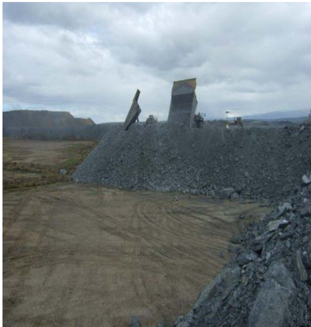
Plate 7. Rock Stack Tip Face (initial lift)
