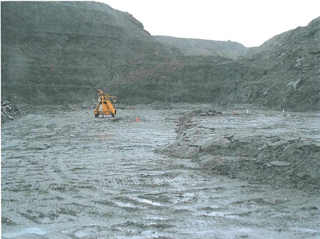
Photo 1: Example of floor heave occurring in the floor of the Frasers pit
