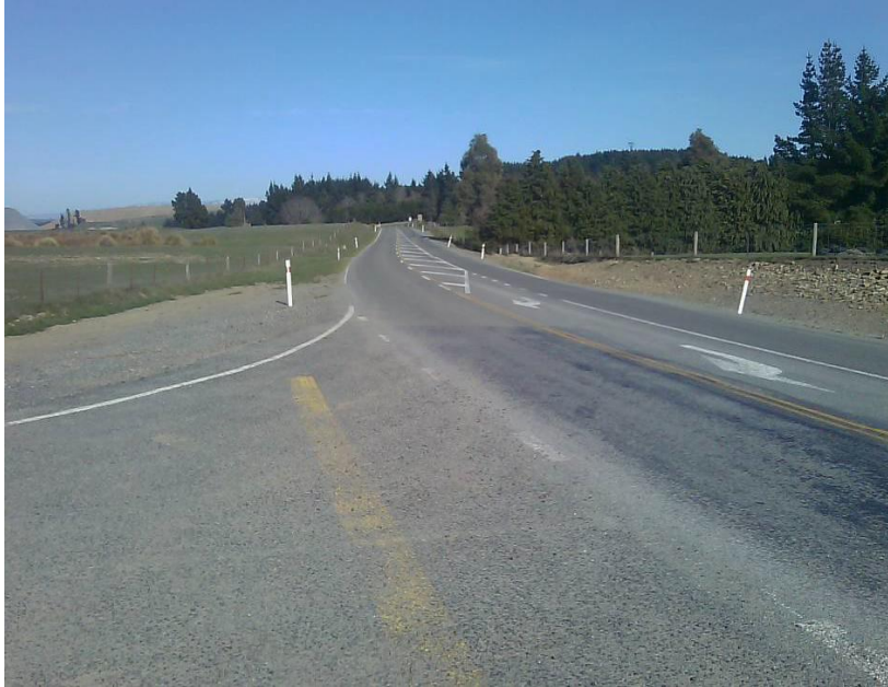
Photograph 5: Right-turn lane at Macraes Road / Golden Bar Road intersection
