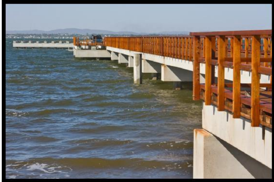
Figure 6 – Completed Moreton Bay Jetty – Substructure and Handrailing
