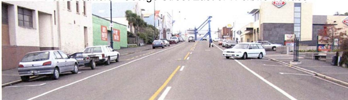
Port Chalmers - George Street East of Wickliffe Terrace
