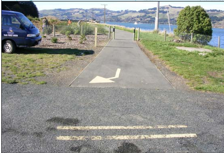
Start of cycleway western side
