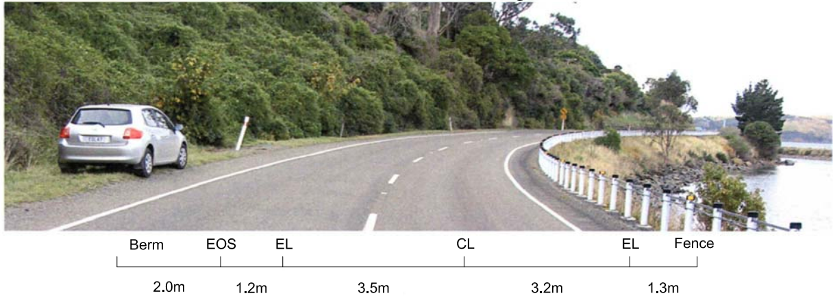
East of Burkes Drive - Looking Eastbound
