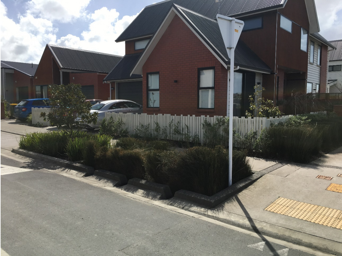
Figure 7: The incorporation of “rain gardens” into a new housing area in Auckland.
