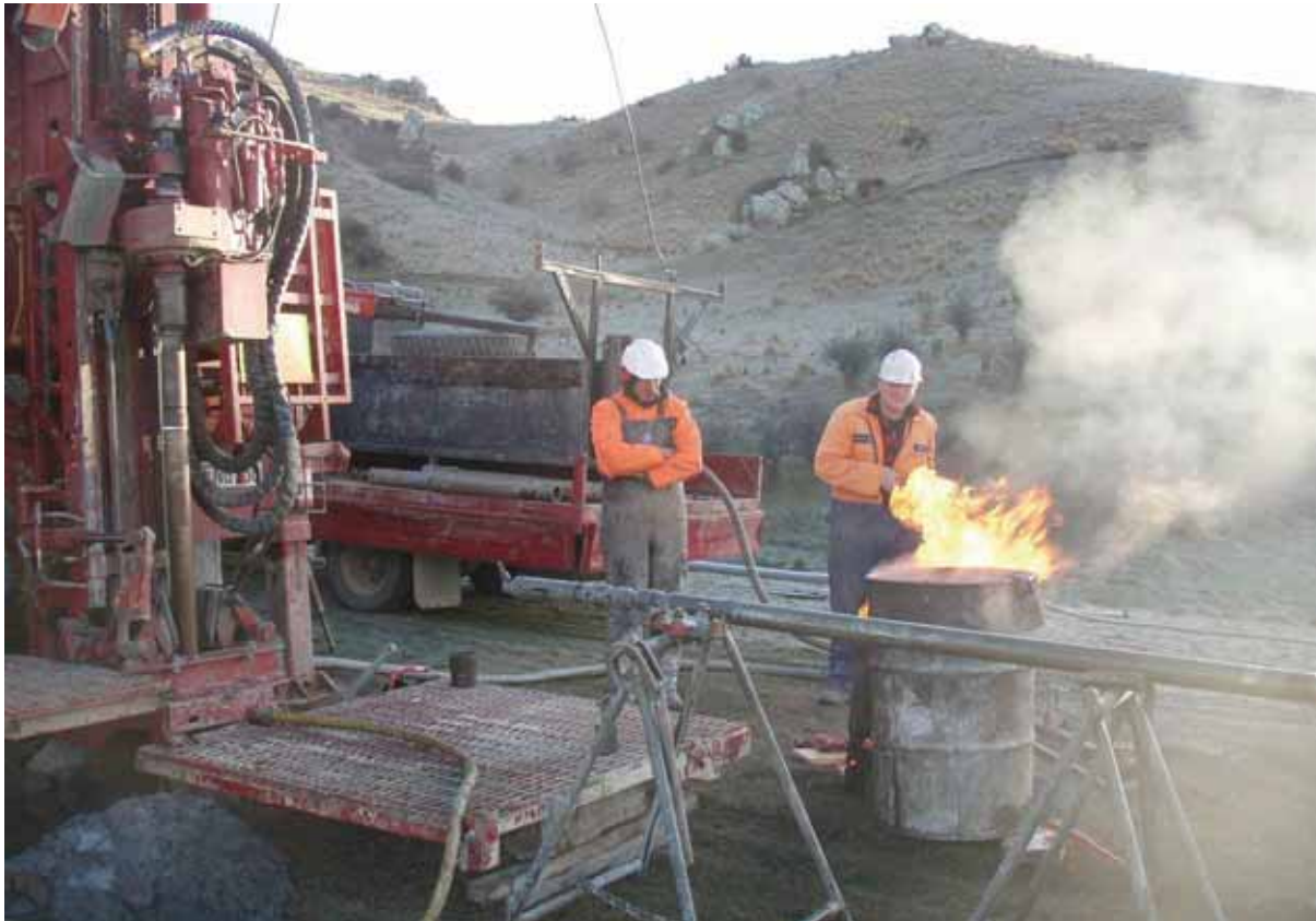
Figure 8. Defrosting while coring in schist at Meade Road.
