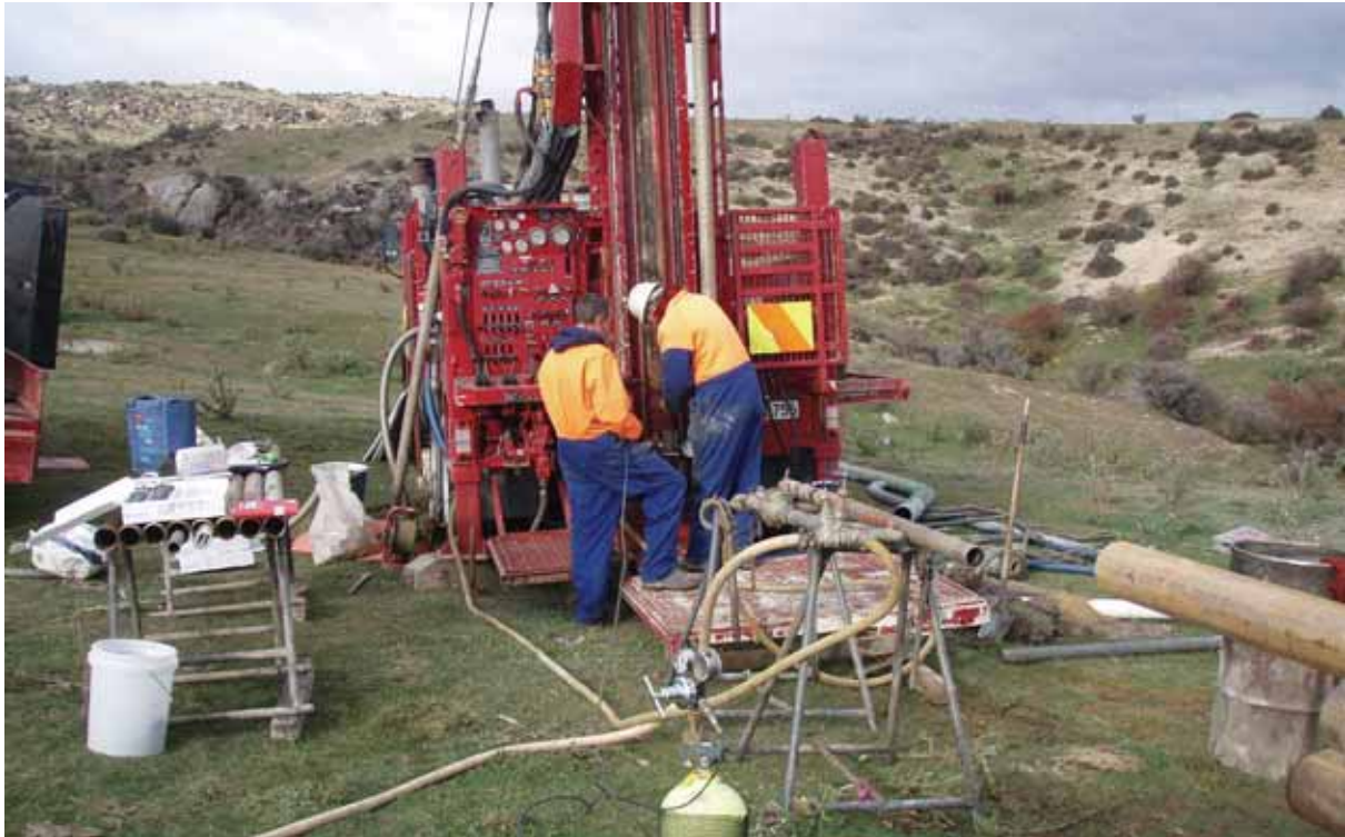
Figure 6. Installing the wireline packer at Cresslea.
