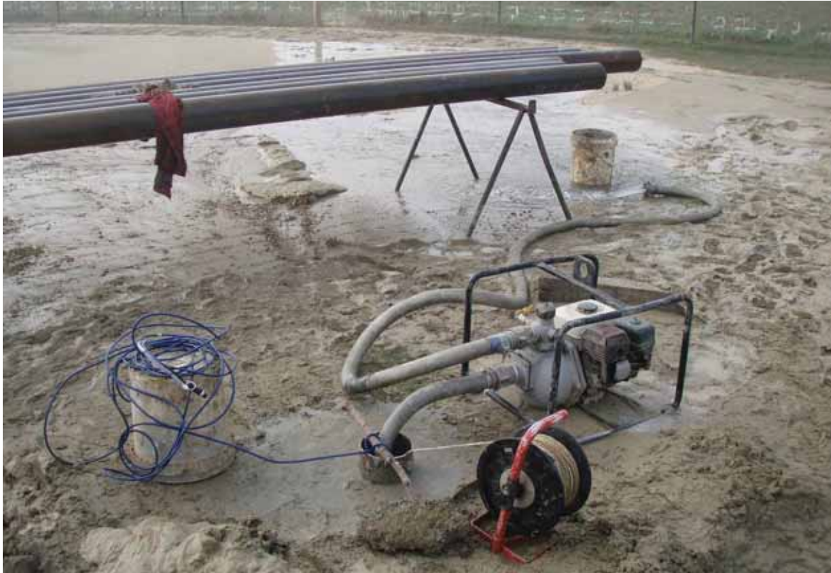
Figure 10. Preliminary pumping test carried out at Meade Road.
