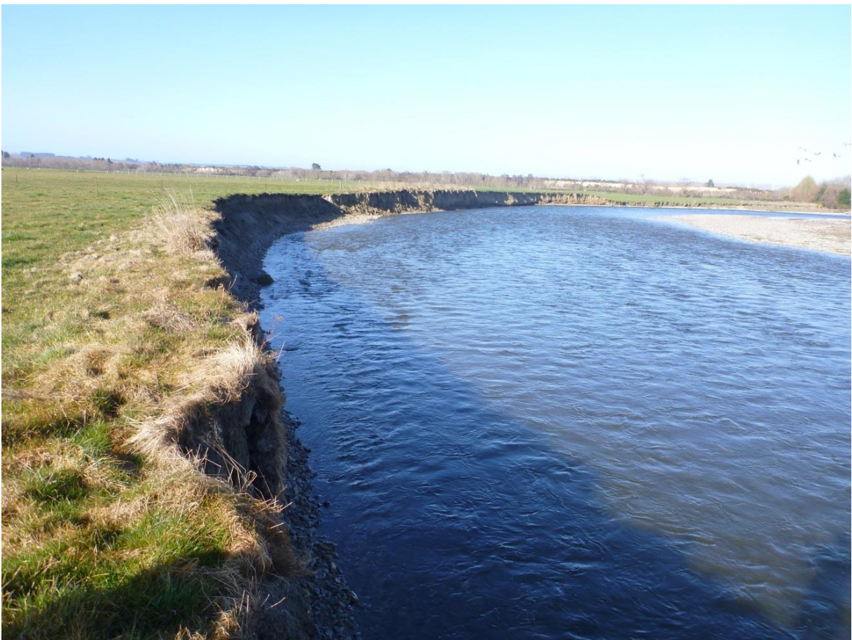
Figure 2. Examples of changes in channel morphology. Top: bank erosion downstream of the Greenvale Road bridge (November 2015); bottom: bank erosion at Camperdown Bend (August 2015)
