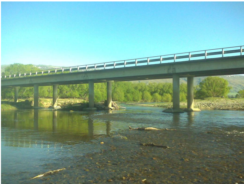
Figure 31. Cross-section ST7, looking upstream, November 2015
