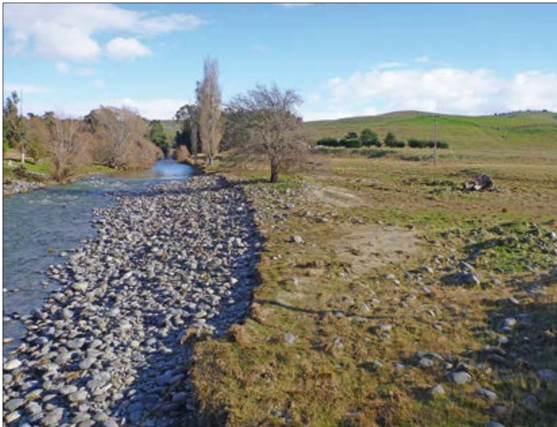
Figure 6. View upstream of Kauru Hill Road bridge (July 2013)
