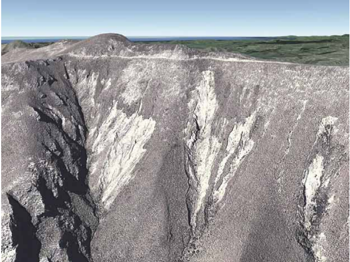
Figure 2. Evidence of land instability in the upper reaches of the North Branch of the Waianakarua River image date June 2012 (Google Earth). This location is shown on Figure 1 (red circle).
