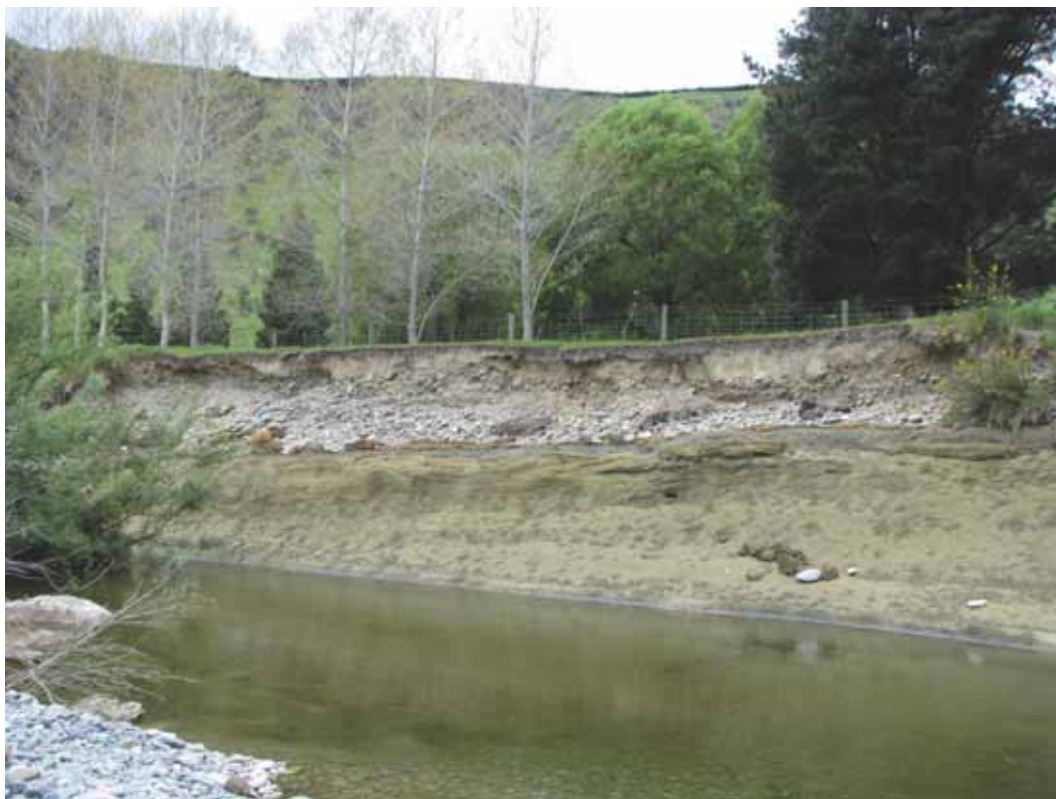
Figure 8. Area of active bank erosion on the North Branch of the Waianakarua River (upstream of SH1), looking upstream, October 2013
