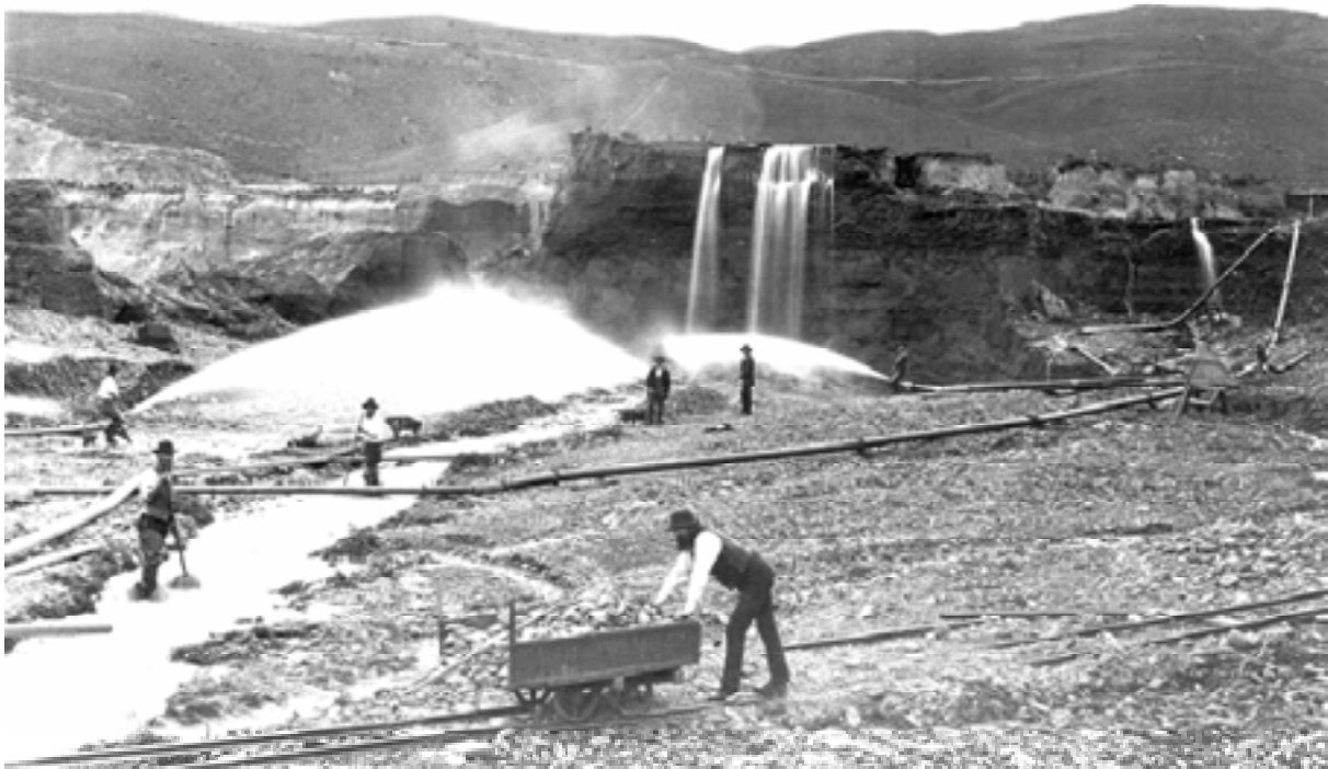
Figure 4.1 Hydraulic sluicing in the Clutha Catchment
