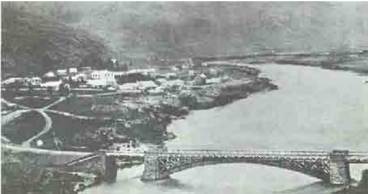
Figure 3.3 Roxburgh bridge in 1875 looking upstream
