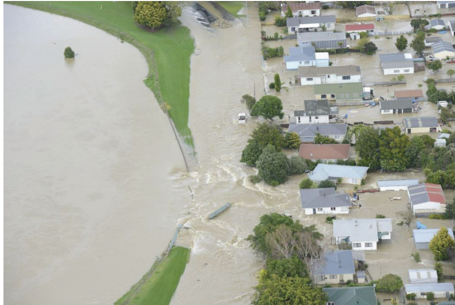
Figure 21: The breached Floodwall at Edgumbe, at 11:00 6 April. Some of the wall sections can be seen still standing upright in the floodwaters some 2.5 hours after the initial breach (Source: Bay of Plenty Regional Council, 2017)
