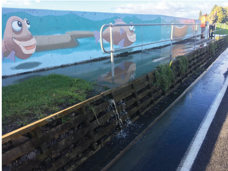
Figure 18: The Edgcumbe Floodwall, known locally as 'The Painted Wall', at 08.14 on 6 April, 15-20minutes before the breach (Source: Bay of Plenty Regional Council, 2017)
