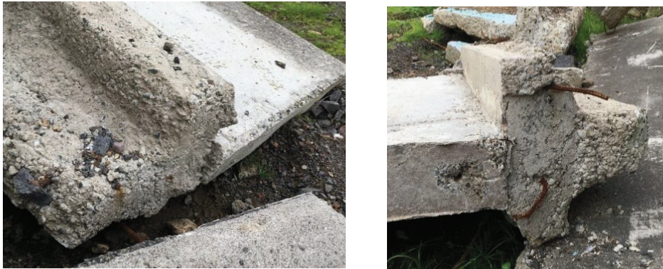
Figure 23: College Road floodwall - Views of the ends of two of the wall sections, showing the subsurface keys (Source: Bay of Plenty Regional Council, 2017)
