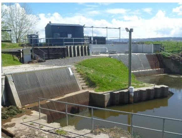
Photo 17: Waipori Pumping Station looking towards Lake Waipori. Pump intake trash racks visible.
