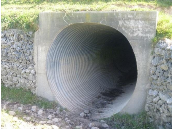
Photo 53: Inlet to the Lower Pond Outlet culvert.
