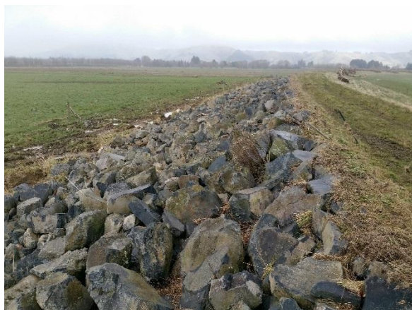
Photo 23: Riverside Road Spillway, long overflow broad crested weir section looking downstream.
