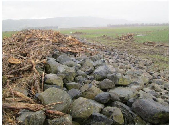
Photo 26: Crest debris from July 2017 flood event.
