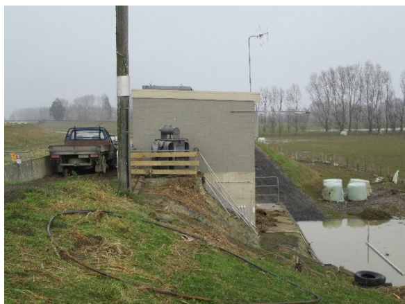
Photo 3: Grouted rock fill below the station transformer and location of historical seepage and seepage reported during July 2017 flood event.
