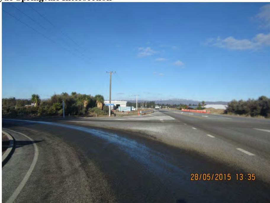
Date: 28/5/15 Description: Stock effluent
