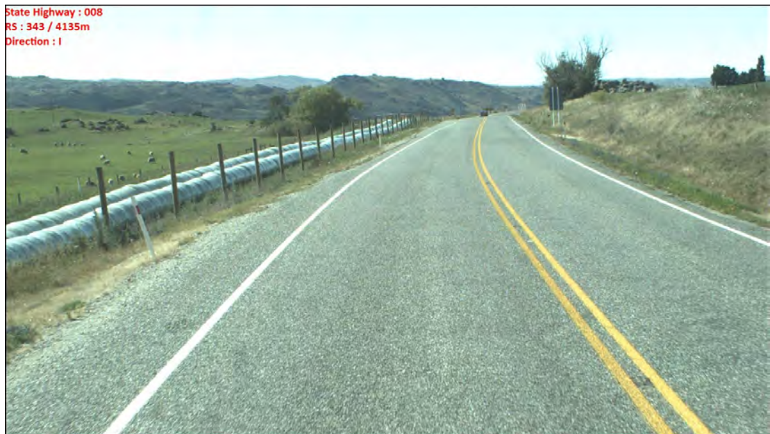
Photo 14: The STED is to be located on the left side of the photo
