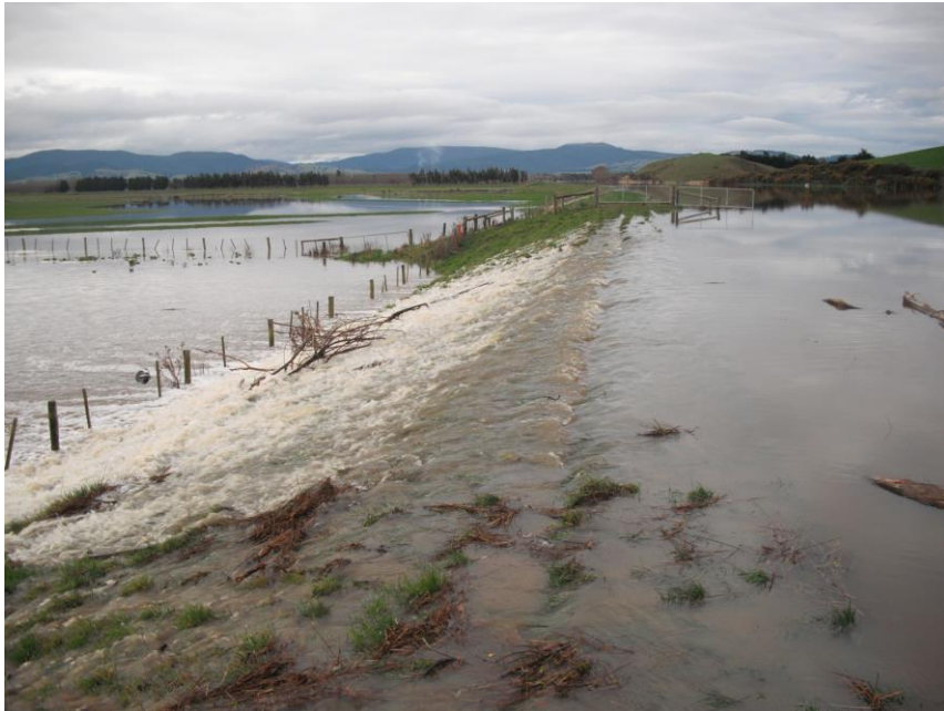
Figure 4.31 Overtopping of the Owhiro Stream into the East Taieri Lower Pond on 15 August, 2012.
