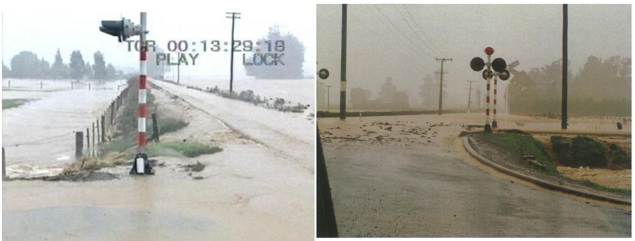
Figure 4.29 Water ponding behind the Taieri Gorge Railway during the April 2006 flood event.
