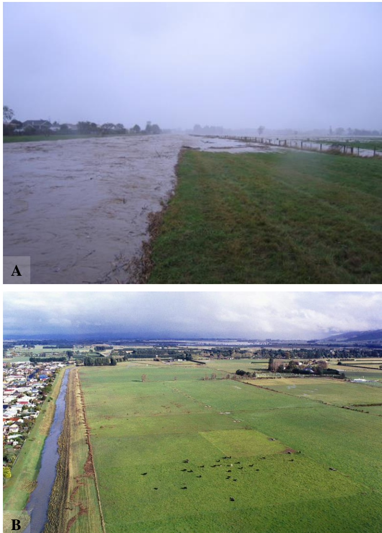
Figure 4.8 Silver Stream flows spilling over the Gordon Road Spillway, 26 April 2006 (A), and Silver Stream looking south (downstream) near Gordon Road on 28 April 2006, with the spillway on the true-right bank (B). Floodwater within the Upper Pond can be seen in the distance.
