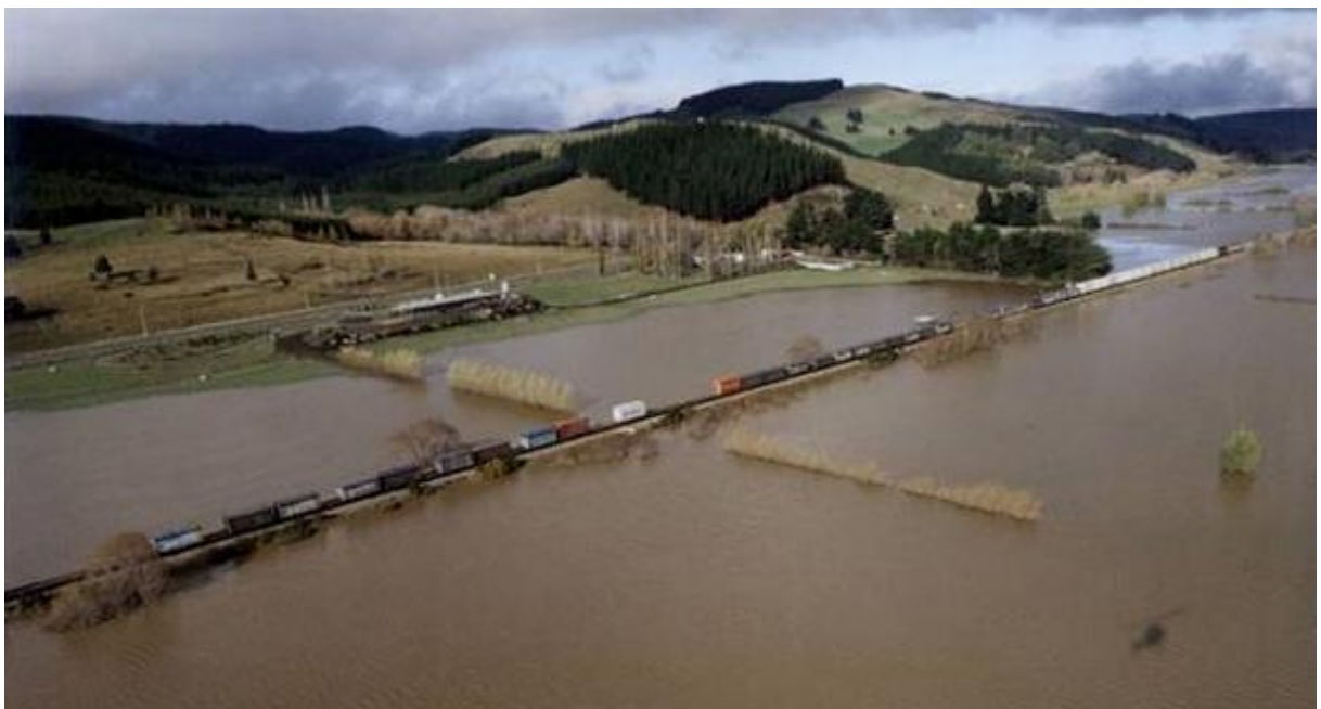
Figure 2.10 South Island Main Trunk Railway, after the April 2006 flood on the Taieri Plains. The south-bound train was forced to stop and wait.
