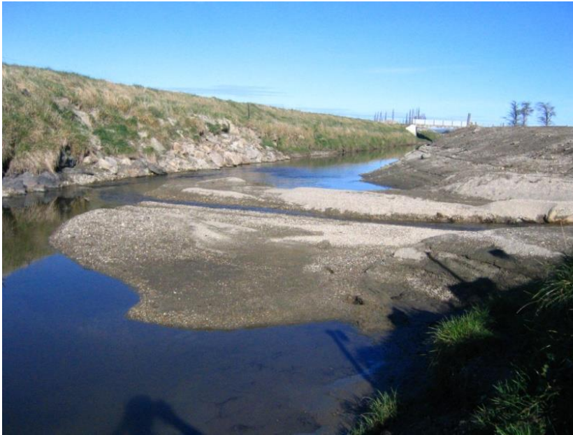
Figure 4.15 Deposition of gravel in the Contour Channel from a tributary hill stream.
