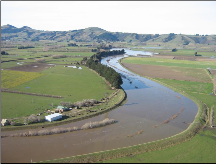
Figure 4.6 Looking downstream towards the chute. The photograph was taken on 31 July 2007, the day after the river peaked at 1,067 m 3 /s at Outram.
