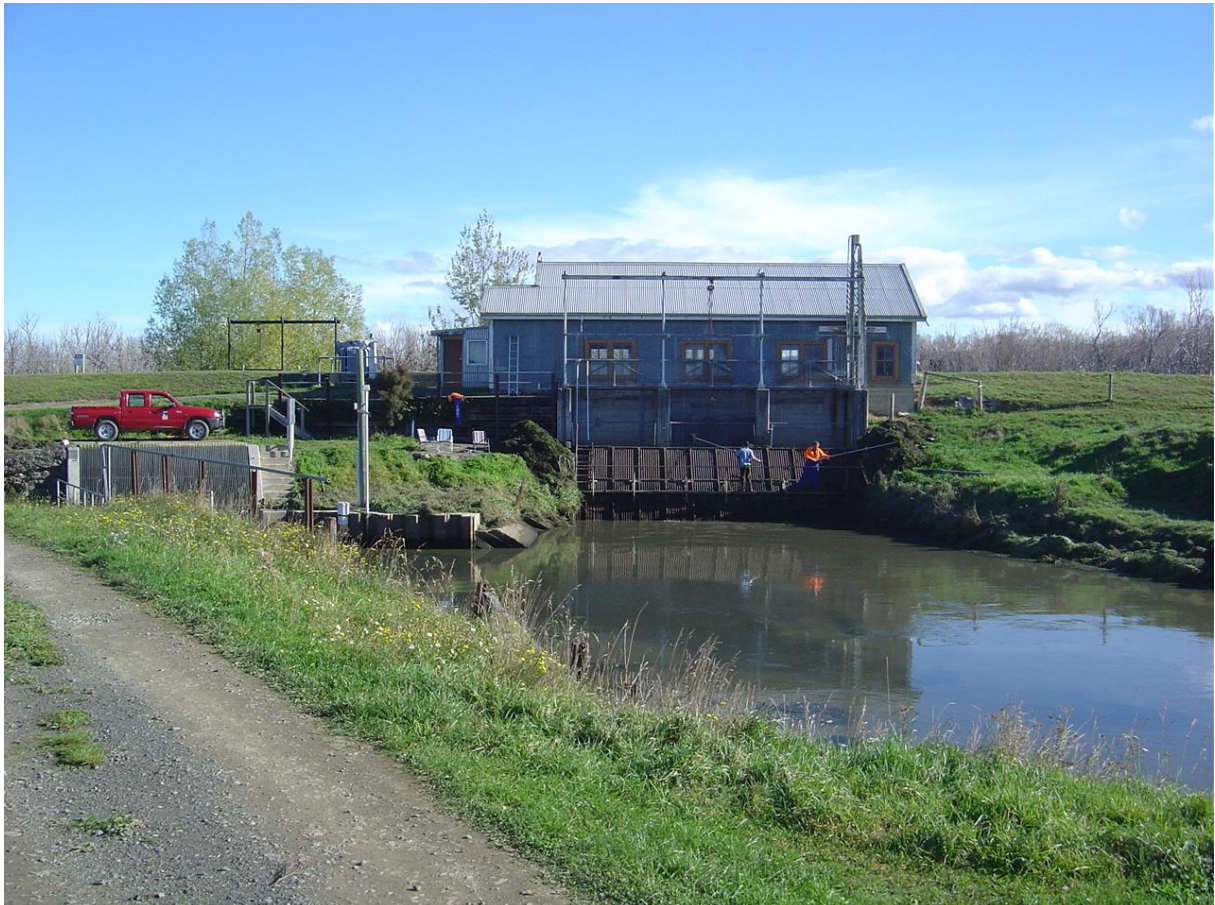
Figure 3.13 Waipori Pump Station and the inlet channel to the station (Main Drain). The underground chamber (installed in 1989) housing the two ‘D’ pumps is on the left, and the building housing the three ‘F’ pumps installed in 1929 is on the right. The three ‘F’ pumps are being replaced with two new submersible pumps in 2012/2013.
