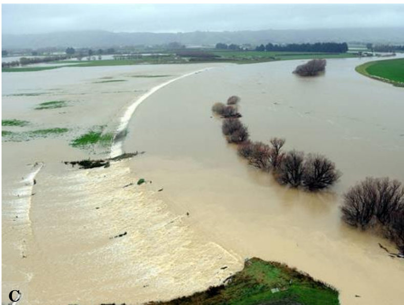
Figure 4.5 Destruction of the Riverside spillway into the Upper Pond after the December 1993 flood (A) Taieri River flows spilling into the Upper Pond on 26 May 2010 (B) and 29 May 2010 (C) over the current spillway. Photos (B) and (C) courtesy of Otago Daily Times.
