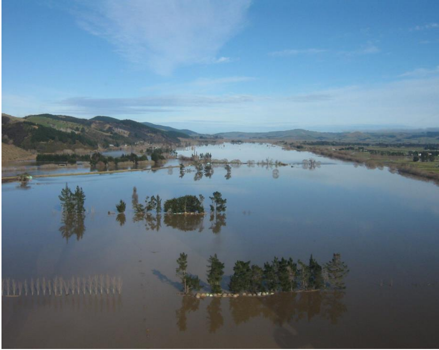
Figure 4.20 Lower Taieri Floodway, looking downstream to Henley, 31 July 2007.
